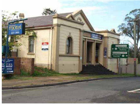
Figure 4: The School of Arts Building, Windsor
