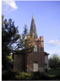
Figure 2: St Peters Anglican Church, Richmond
