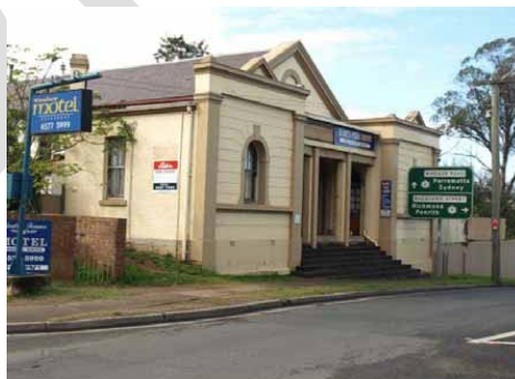
Figure 4: The School of Arts Building, Windsor
