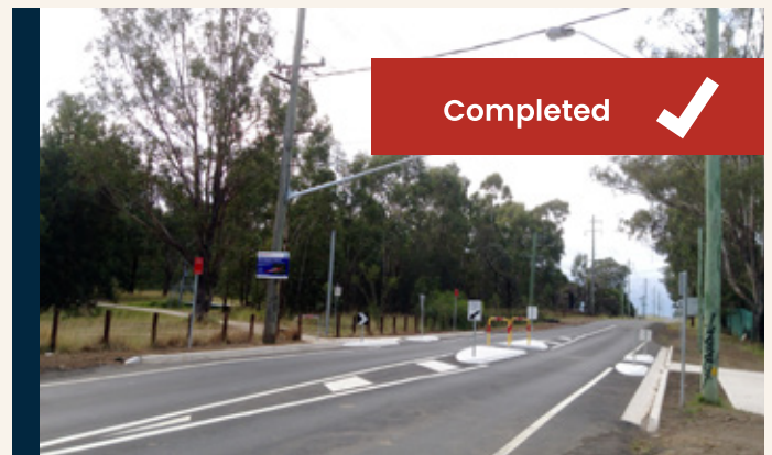
ROAD UPGRADE Berger Road, South Windsor
