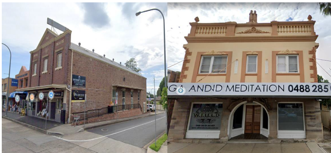
Figure 24 – Architectural Roof Feature within Hawkesbury’s Town Centres
