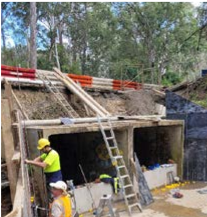
Reconstruction of Valley Way at Tennyson, including new drainage culvert
