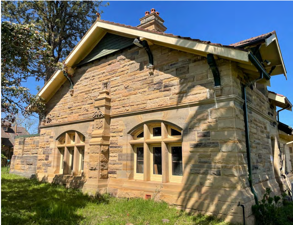
Plate 3-21: North eastern elevation with carved finial with "1896", identical to Building 1 (AECOM, 2022)
