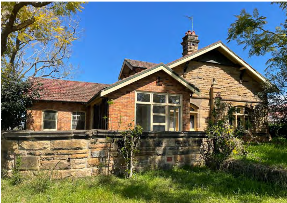
Plate 3-9: North eastern elevation of Building 1. Note commemorative stone in retaining wall at lower left (AECOM, 2022)
