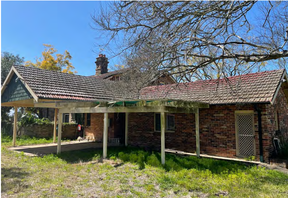
Plate 3-11: Modern portico (left) and addition (right) to Building 1 (AECOM, 2022)
