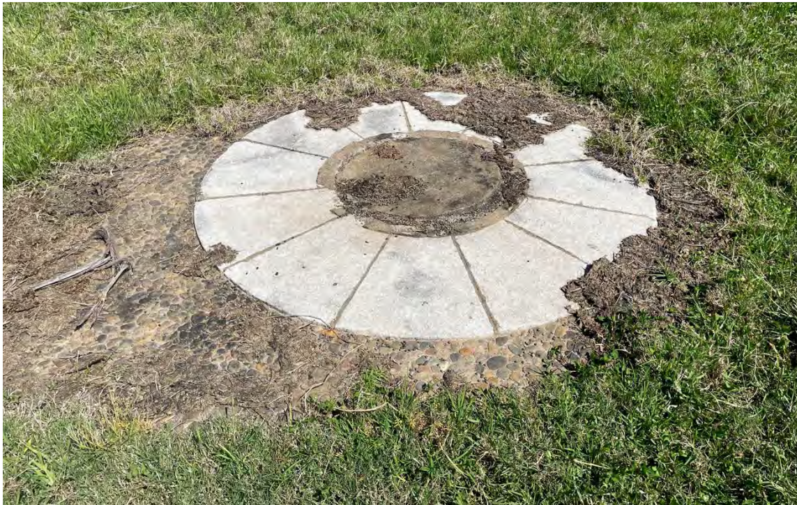
Plate 3-19: Portion of pebbled path and foundation (AECOM, 2022)
