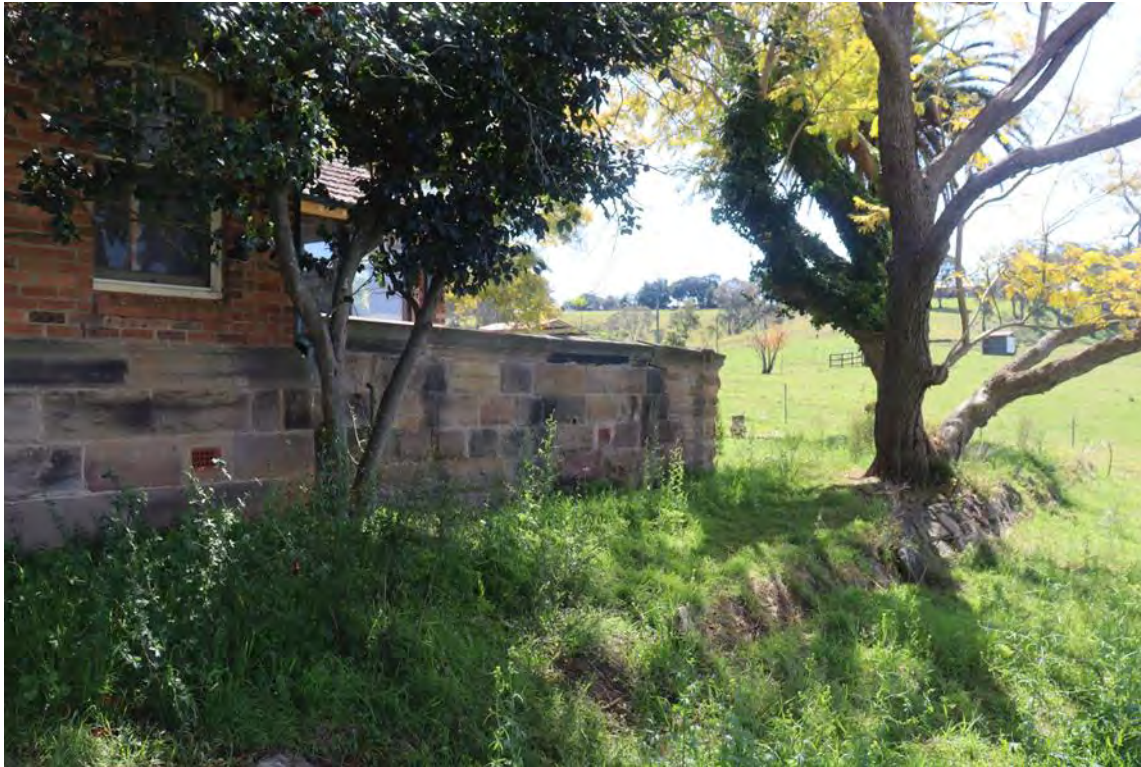
Plate 3-12: View north of the curved retaining wall (AECOM, 2022)
