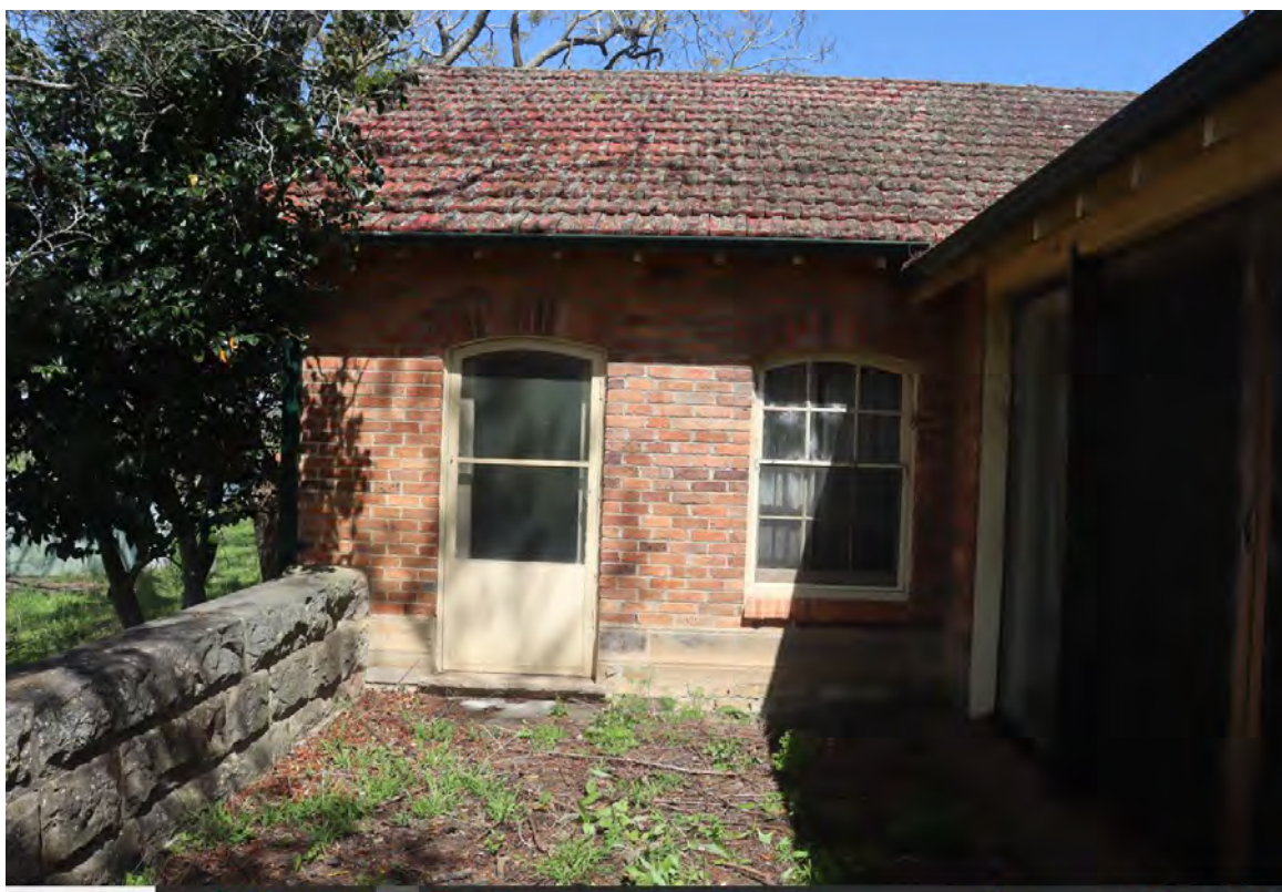
Plate 3-10: Brick addition to Building 1 at north east, however, note stone coping and wooden window and door (AECOM, 2022)
