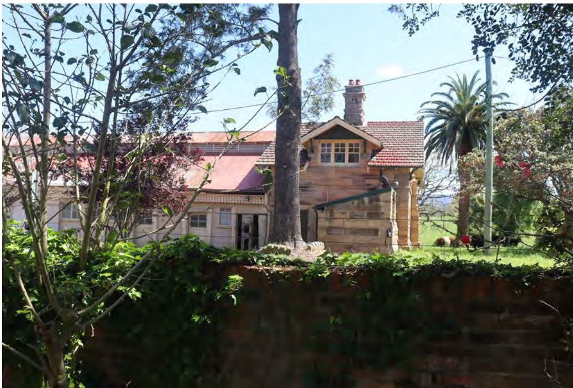
Plate 3-17: View south from garden wall of Building 1 to Building 2 (AECOM, 2022)
