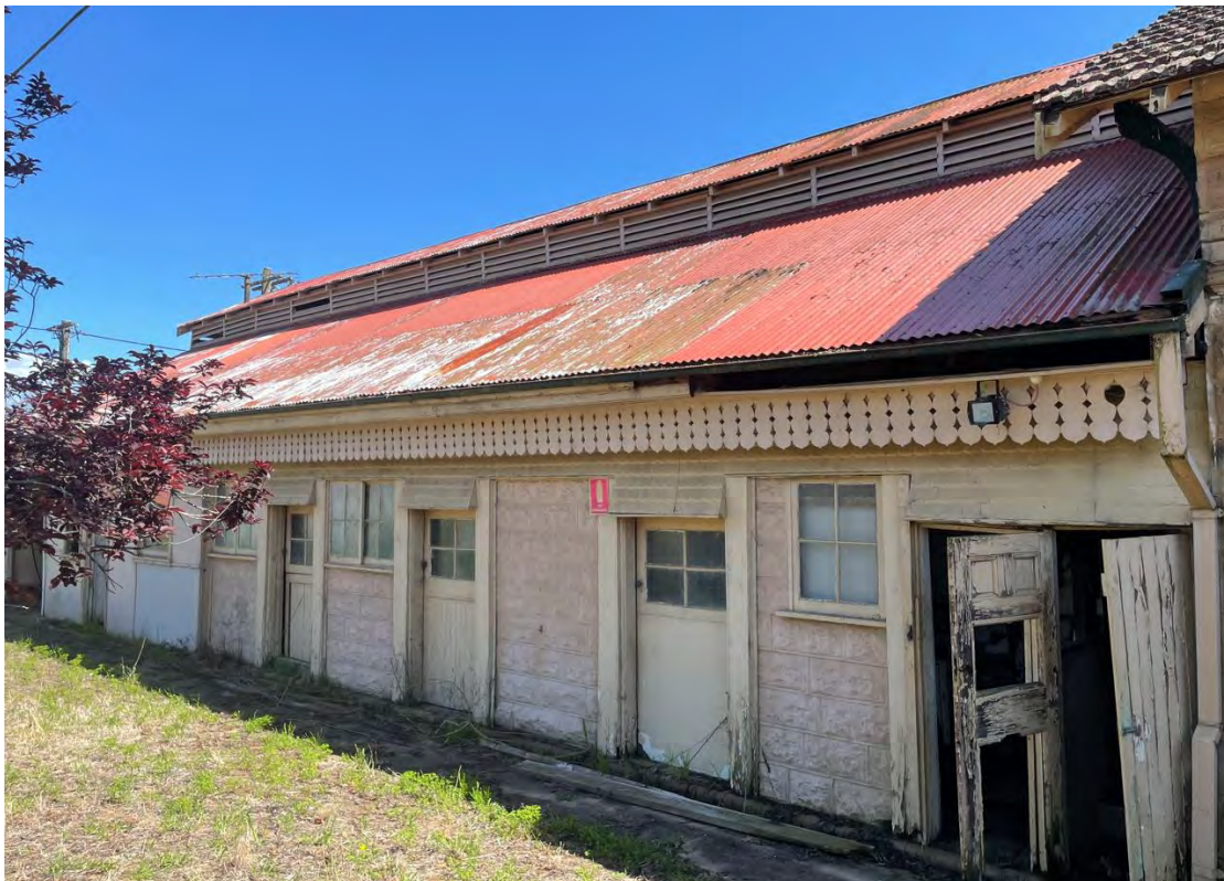
Plate 3-22: South-eastern elevation of Building 2 (AECOM, 2022)
