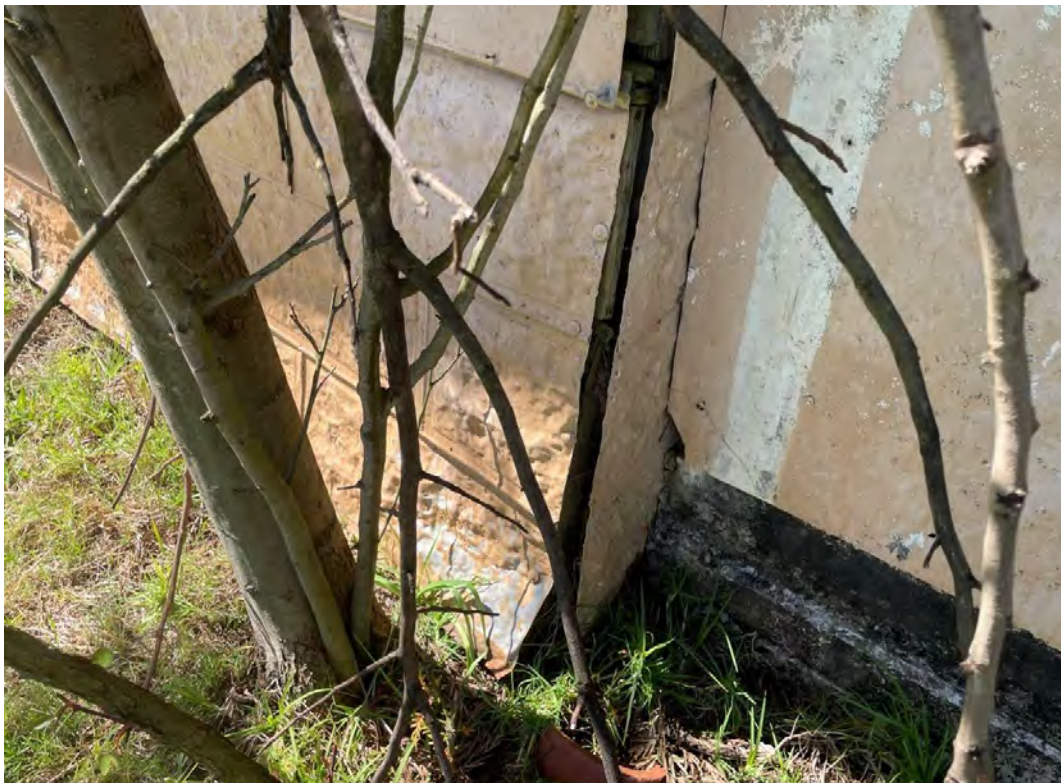
Plate 3-24: Detail of pressed tin cladding with ashlar pattern on external walls of Building 2 (AECOM, 2022)
