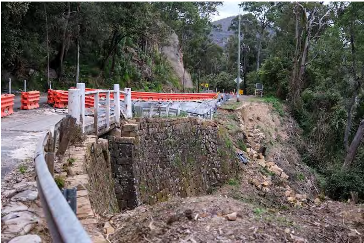
Figure 2-8: View of landslip to embankment at Thomas James Bridge. Source: ABC News, https://www.abc.net.au/news/2022-10-21/hawkesbury-community-limited-access-drinking-water-after-floods/101540984 21/10/2022
