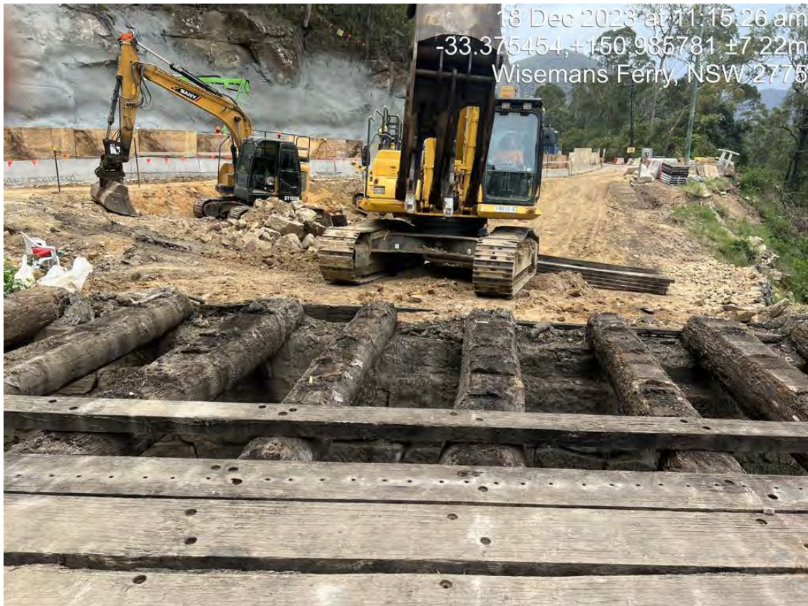
Figure 2-15; Deconstruction of bridge ahead of reconstruction works, showing timber deck. Source: Hawkesbury City Council, 2023.
