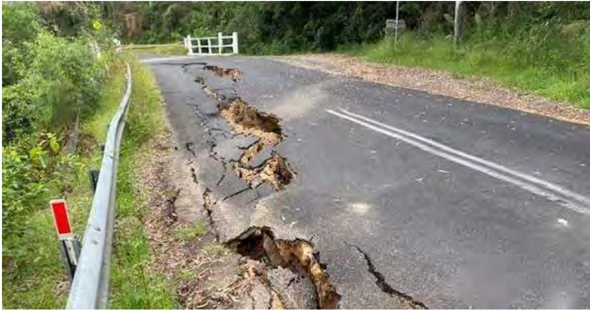
Figure 2-7: Damage to bridge and approach resulting from flooding and resultant landslip. Source: Hills to Hawkesbury , 16/5/2022
