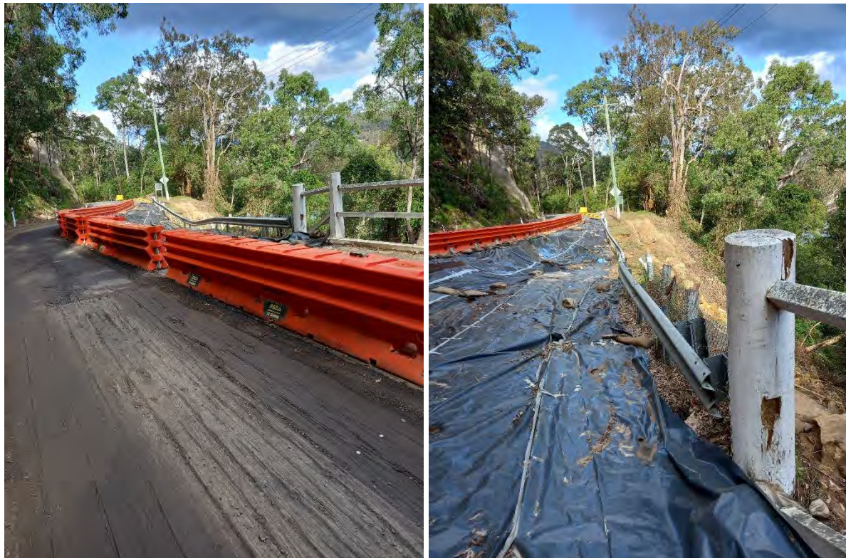
Figure 3-10: Views of the surface of the bridge looking east, with the collapsed section of the slope visible to right. (Source: OCP Architects, August 2022.)
