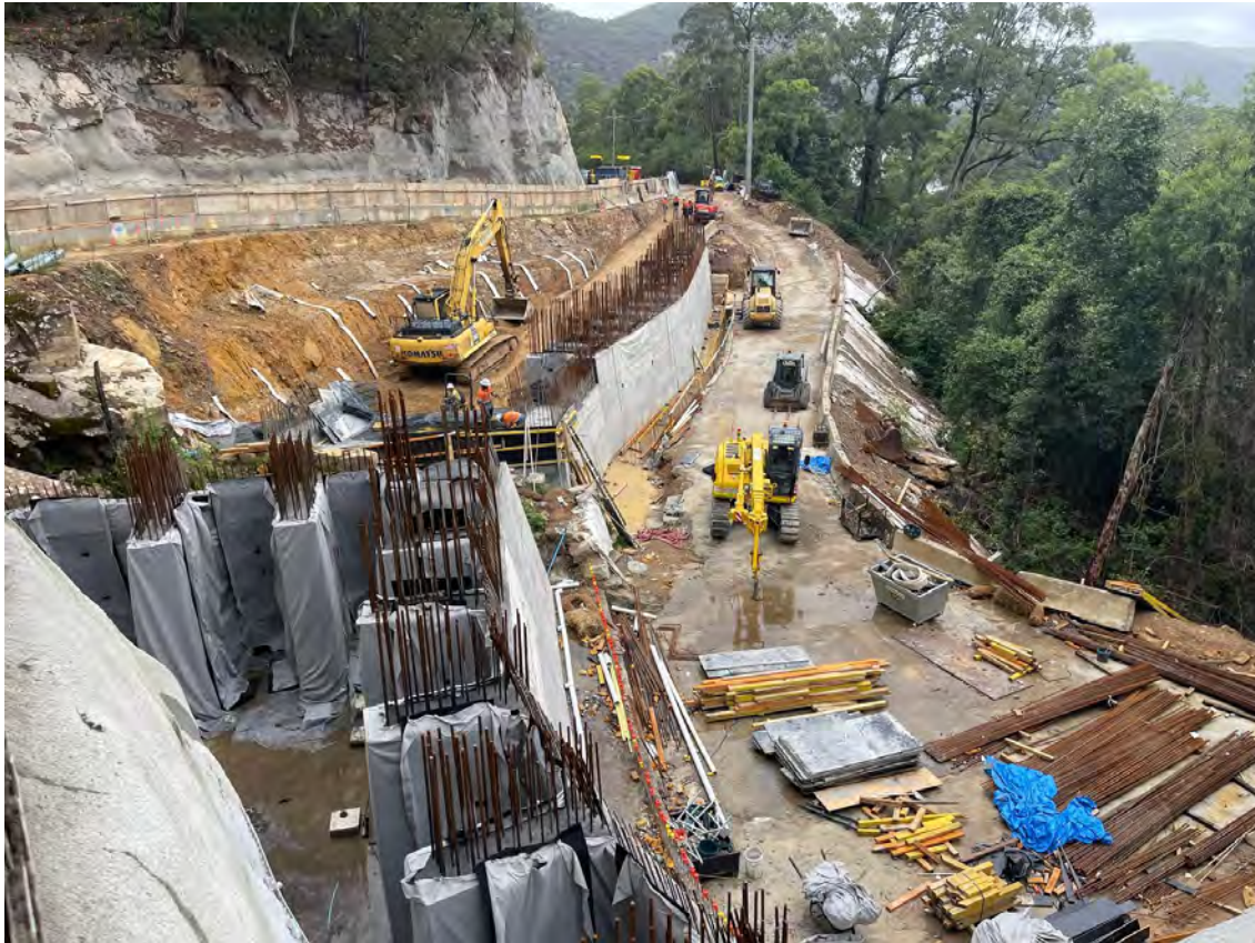
Figure 2-17: Backfilling behind retaining wall during construction works in 2024. Source: Hawkesbury City Council.
