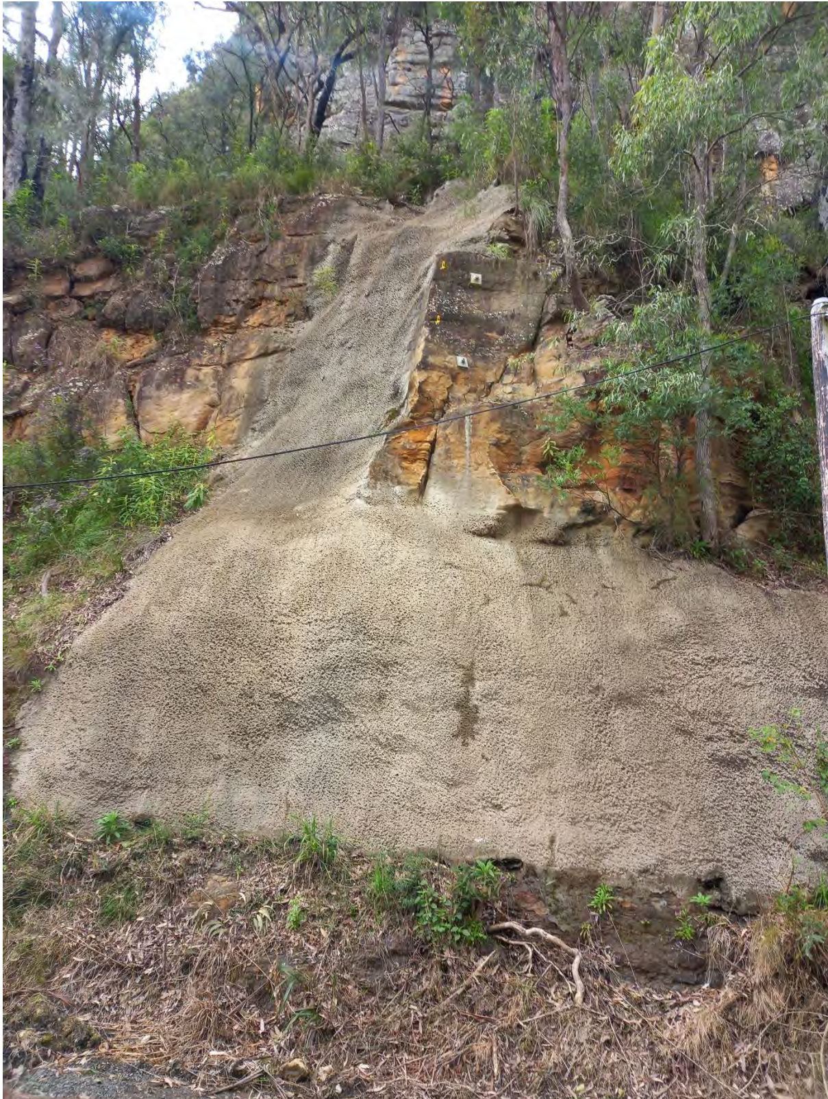
Figure 3-22: View of an existing instance of shotcrete to the escarpment above Thomas James Bridge. (Source: OCP Architects, August 2022.)
