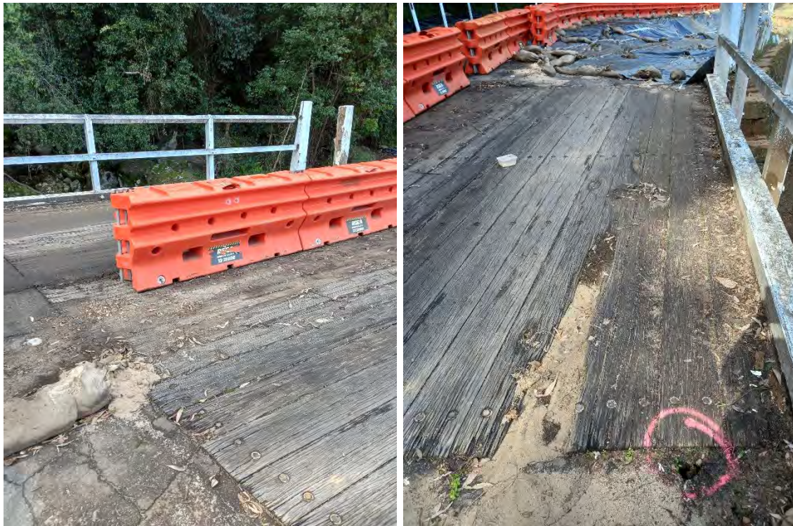
Figure 3-11: Views of the timber decking to the surface of the bridge. (Source: OCP Architects, August 2022.)
