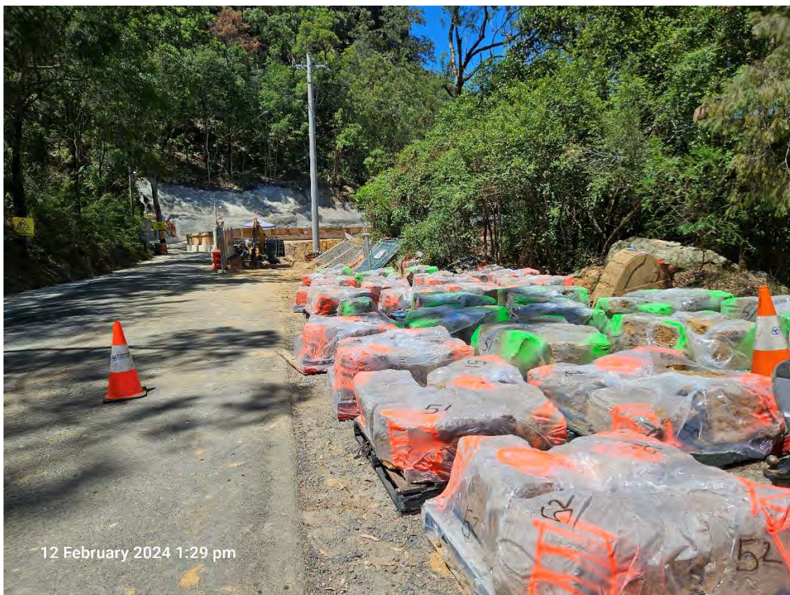
Figure 2-16: Numbering and storing sandstone blocks. Source: Hawkesbury City Council, 2023.
