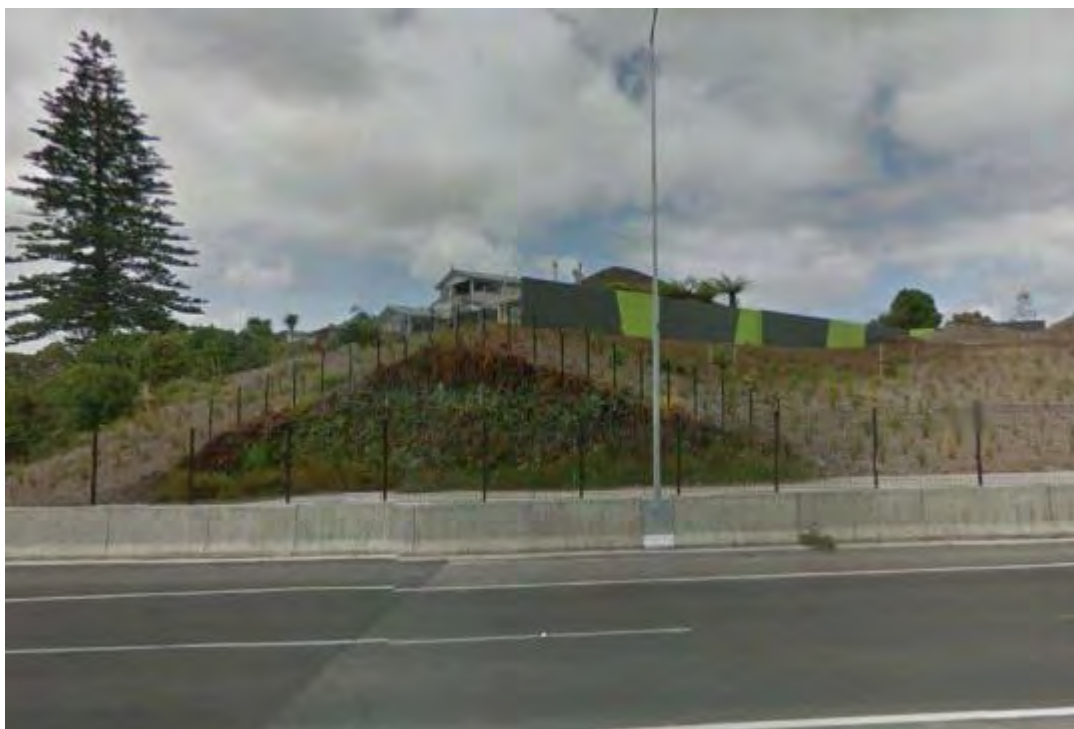
Figure 8-4: Embankment stabilised with shotcrete but finished with vegetation. In this case, the vegetation is not yet mature. (Source: Sydney Trains.)
