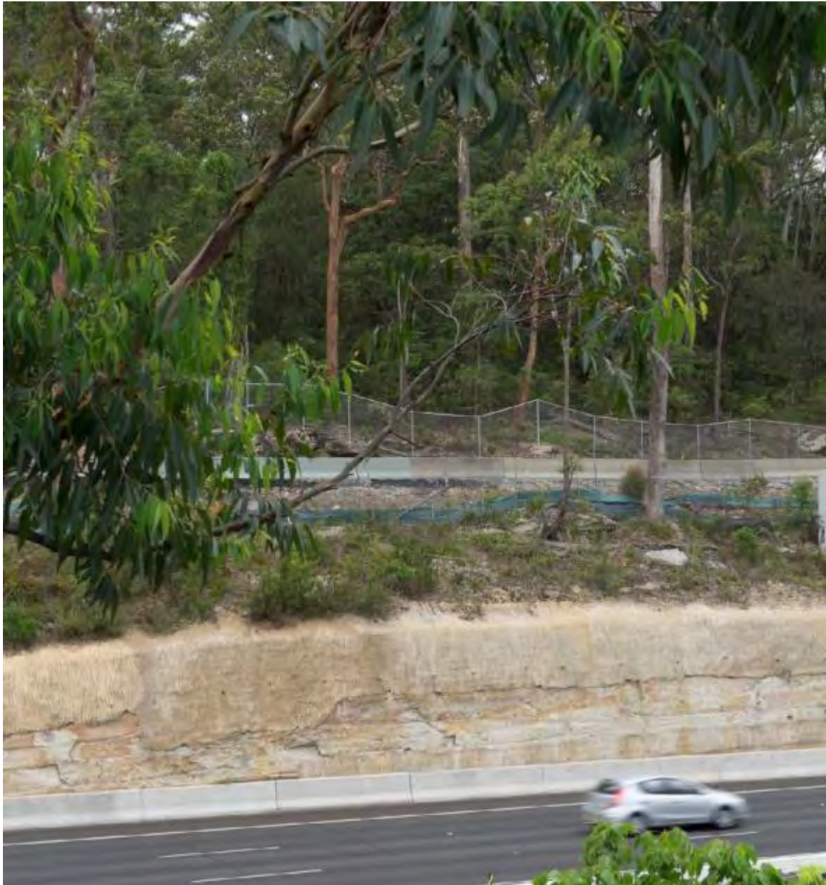
Figure 8-1: Example of shotcrete application with an unobtrusive outcome – in this case (on the M2 upgrade) using ‘cat’s claw’ technique to provide a texture and an oxide applied to the concrete to match sandstone. (Source: RMS Shotcrete Design Guideline.)
