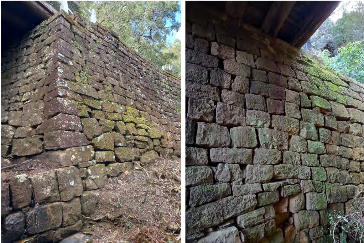
Figure 3-20: Views of the convict-quarried stonework. (Source: OCP Architects, August 2022.)
