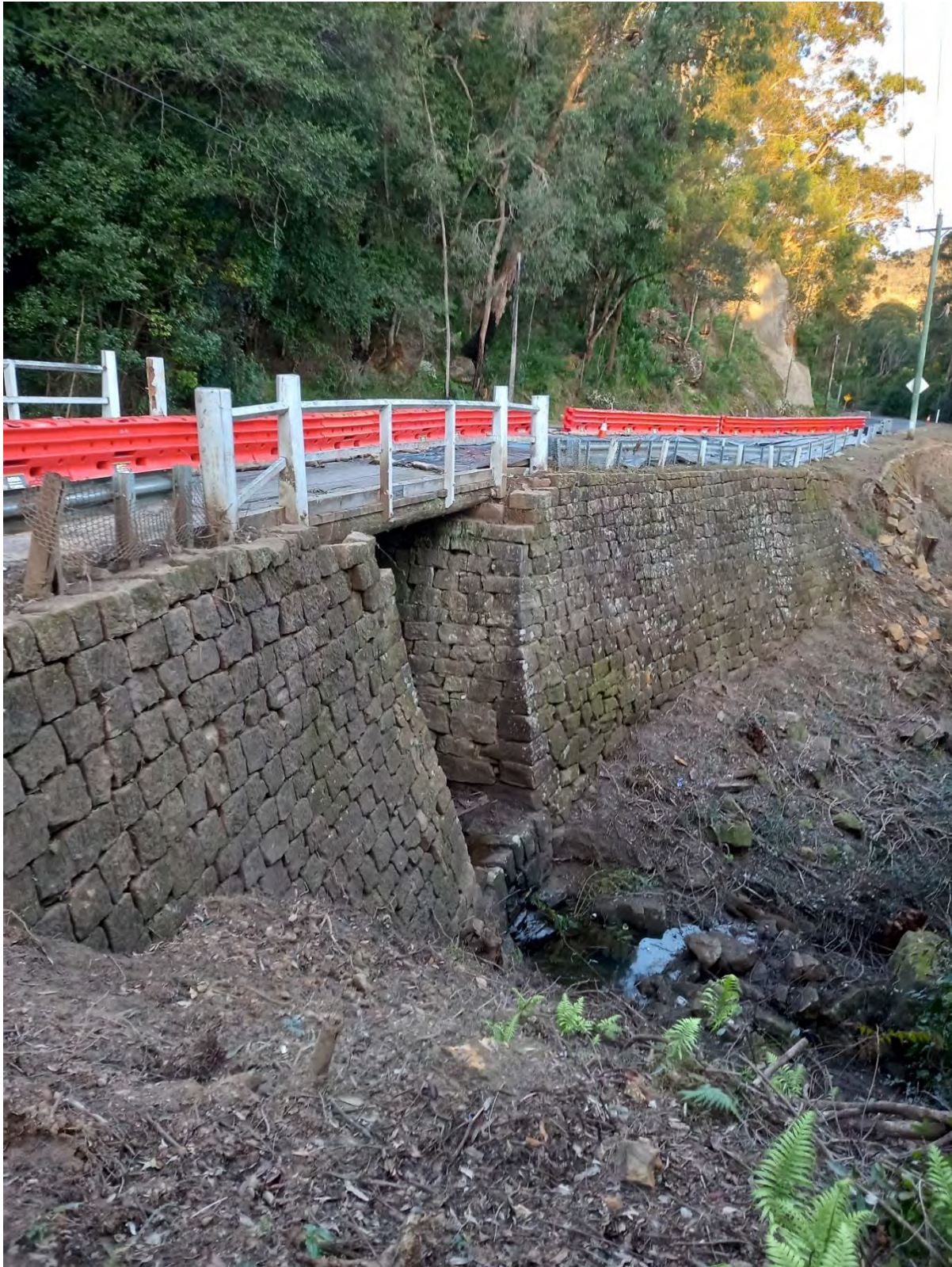
Figure 3-12: View of the bridge and stone abutments on the riverside. A collapsed section of slope can be seen at top right. (Source: OCP Architects, 2022.)
