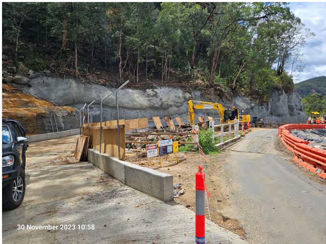
Figure 2-14: Construction of temporary bypass road, 2023. Source: Hawkesbury City Council.
