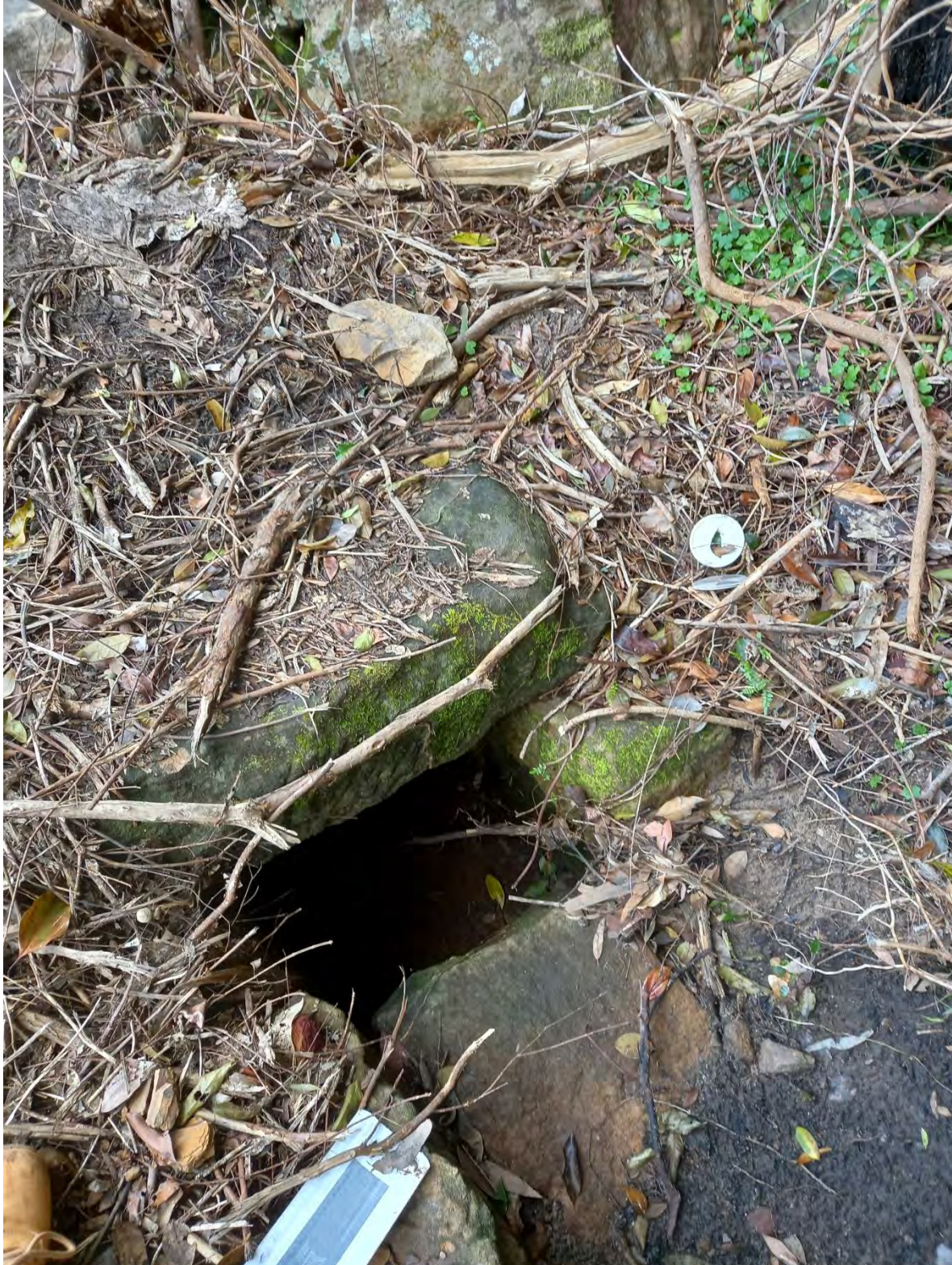
Figure 3-17: View of drainage channel intake. (Source: OCP Architects, August 2022.)
