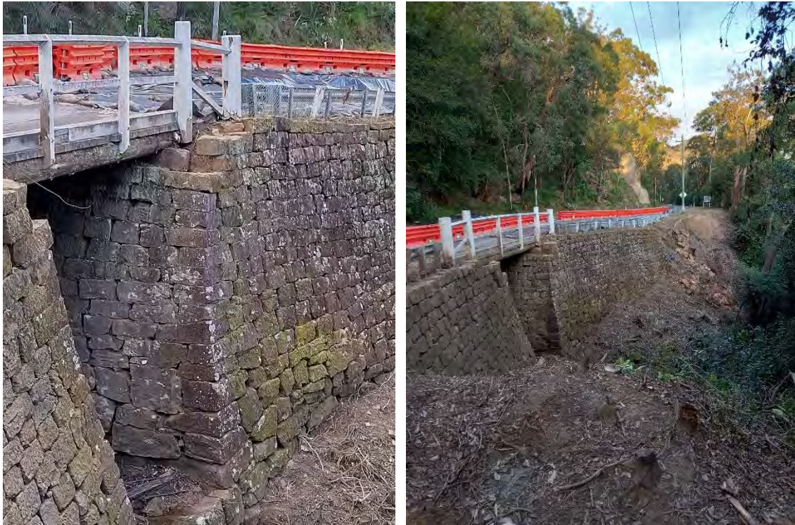
Figure 3-7: View of riverside of Thomas James Bridge, showing convict-quarried stone abutments. (Source: OCP Architects, 2022.)
