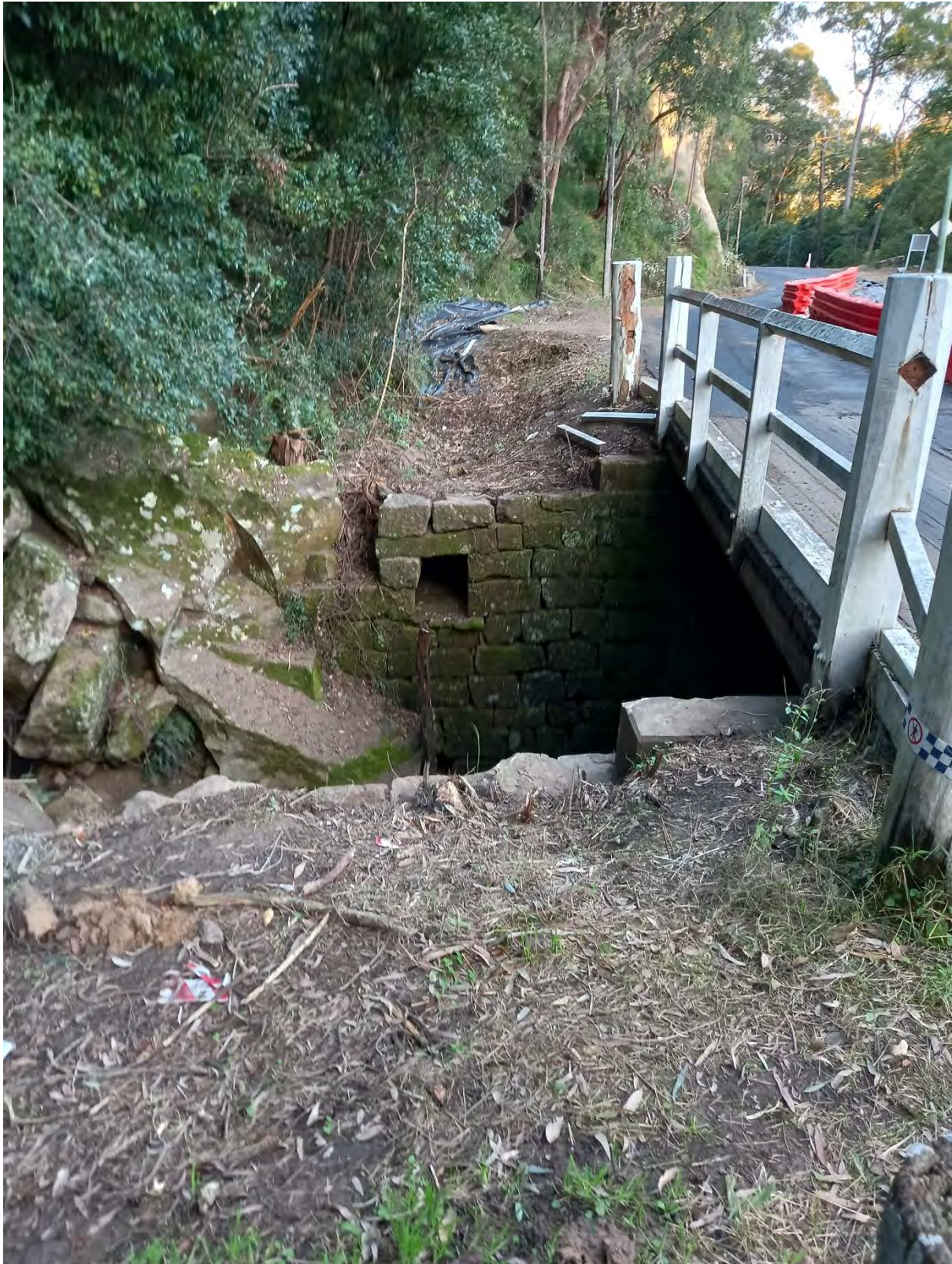
Figure 3-16: View of the bridge to Dharug National Park side, with a drainage channel visible in the face of the stonework. (Source: OCP Architects, 2022.)
