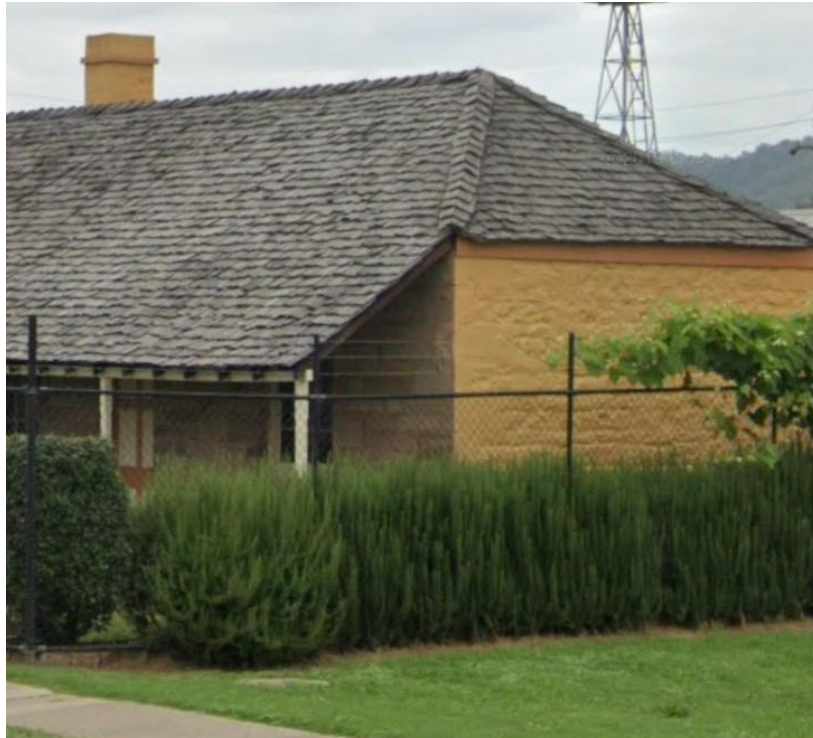
Example of a timber shingle roof, Arms of Australia Inn, Emu Plains
