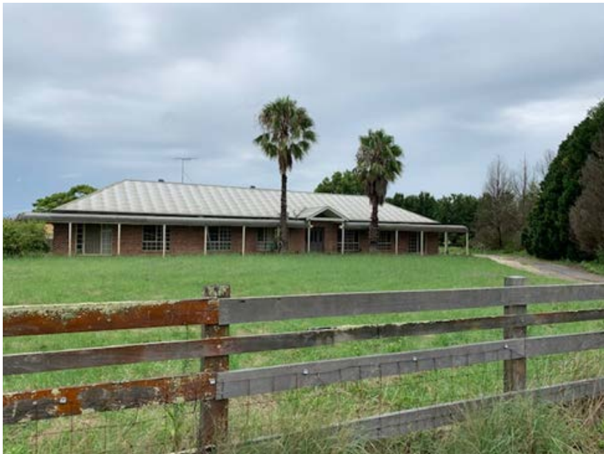
Figure 2: The site contains an existing dwelling house and rear farm building
