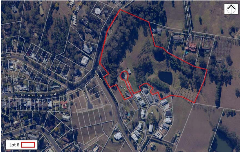
Figure 5: Aerial View of the Subject Site
