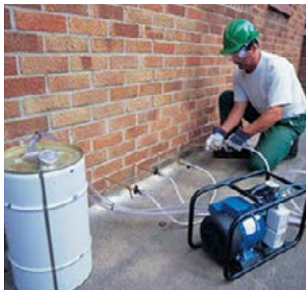
Figure 14: Chemical DPC impregnation in progress
