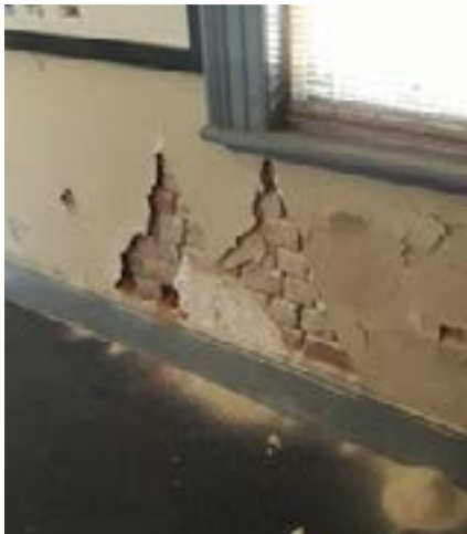
Figure 1: Typical blistering of paint and damage to plaster finish caused by combination of rising damp and salt
