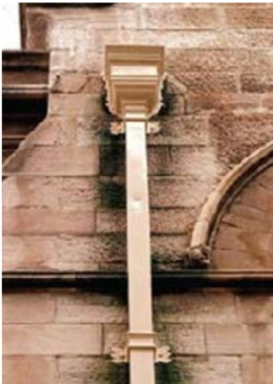
Figure 8: Open joints in cornice stones has allowed water with salts to discolour and damage stonework below
