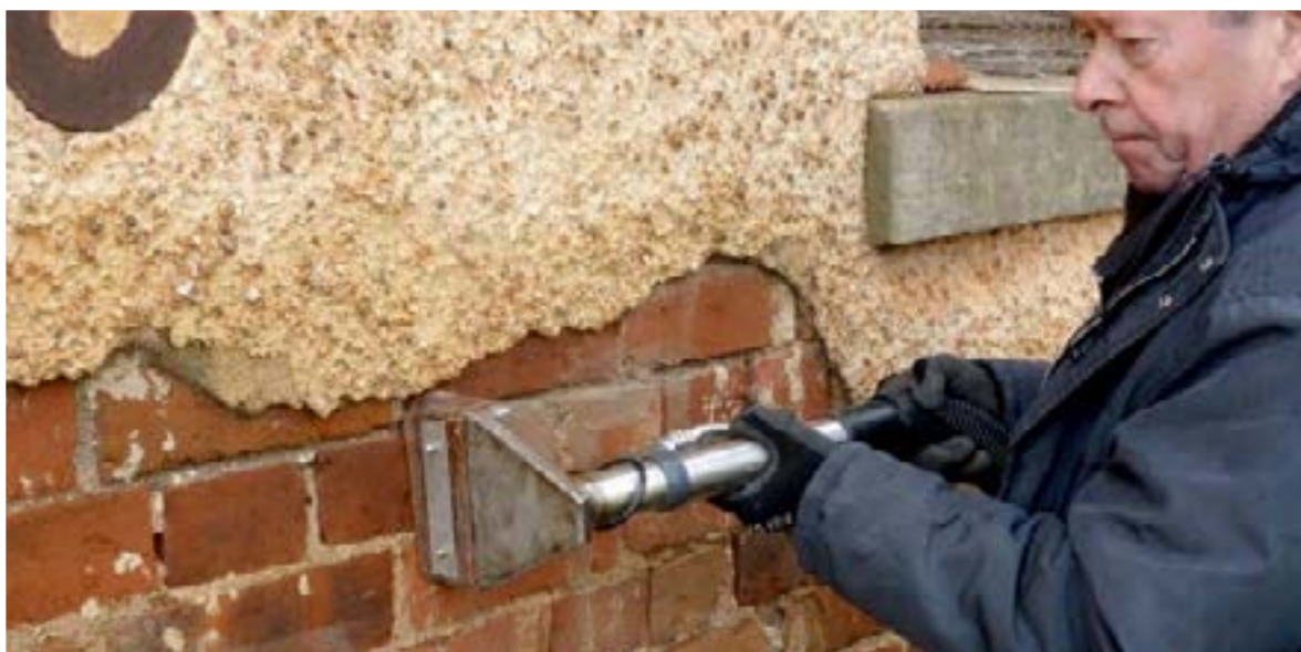
Figure 12: Captive-head vacuum washing
