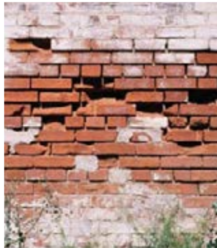
Figure 2: Typical salt damp damage causing decay of the bricks (Heritage Council NSW)
