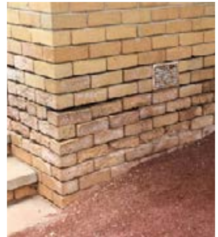
Figure 3: Loss of mortar in joints due to salt attack causing dislodgement of bricks, with white
