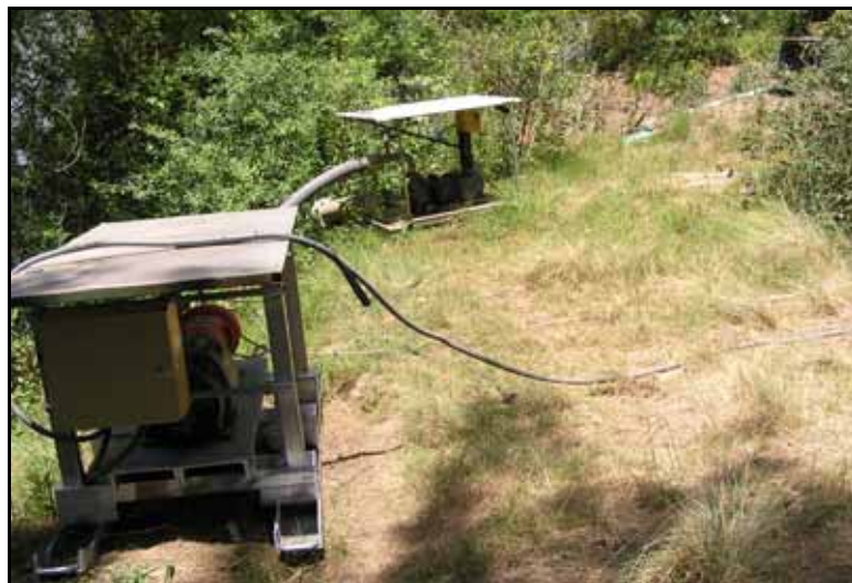
PHOTO 13: The southern portion of the reserve (river bank) contains a number of irrigation pump-sites and piping, overground electrical cabling and unsecured meter boxes on elevated towers. This infrastructure, currently under licence or permissive occupancy on the Crown reserve, raises issues over public safety and risk management. These issues need to be addressed in accordance with this plan of management.
