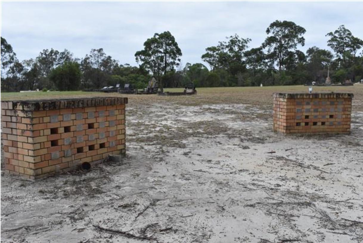
Figure 5 Two brick columbaria situated at the entrance. (Source: GML Heritage, 2019)
