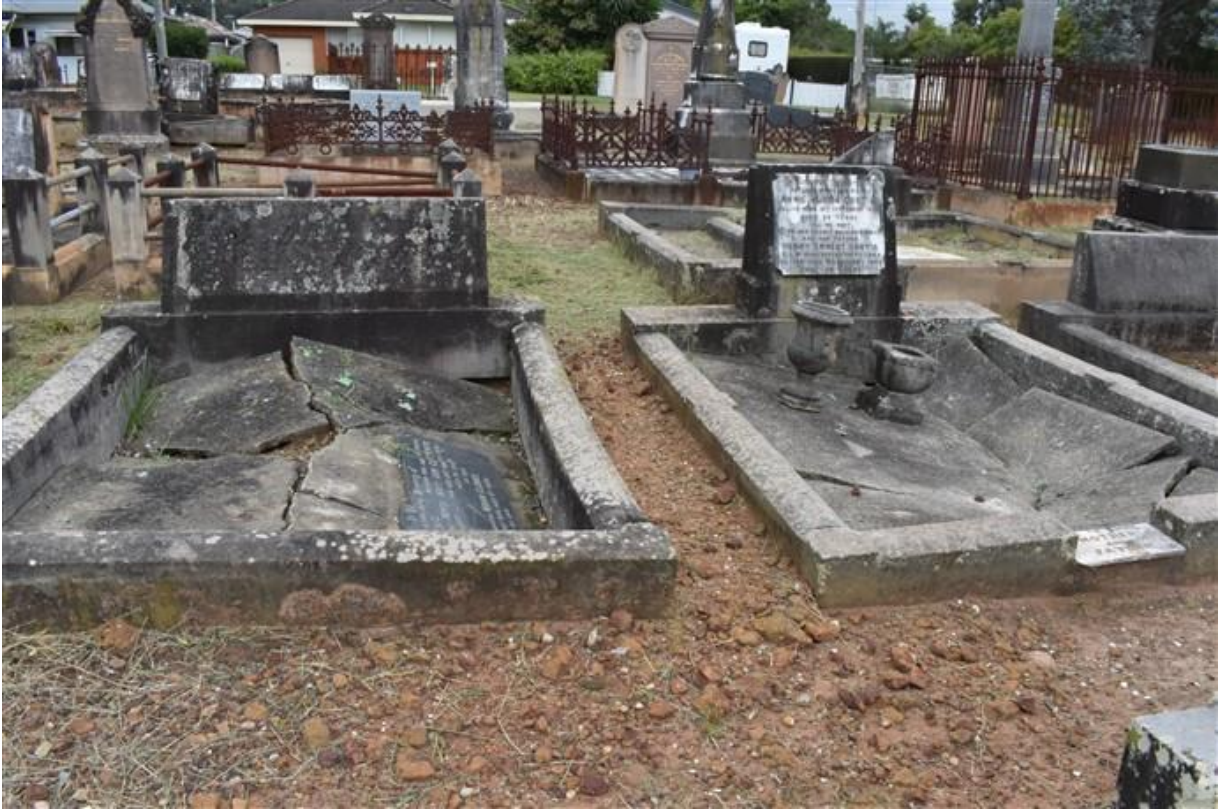
Figure 11 Examples of natural subsidence within burial plots. (Source: GML Heritage, 2019)
