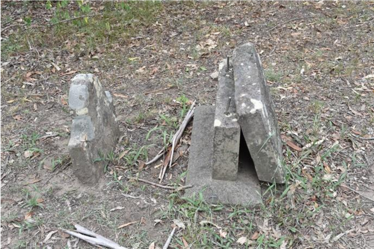
Figure 9 Evidence of previous restoration projects. (Source: GML Heritage, 2019)
