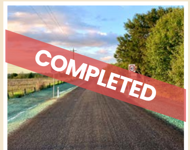
Road rehabilitation at Cupitts Lane, Cornwallis
