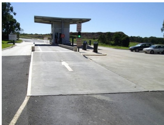
Weighbridges at the Hawkesbury Waste Management Facility
