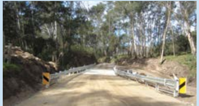
Upgrade on Bridge Number 7 on Upper Colo Road is now complete.
