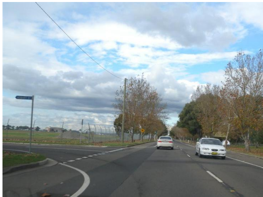
Figure 5.8: Unsatisfactory Intersection Linemarking
