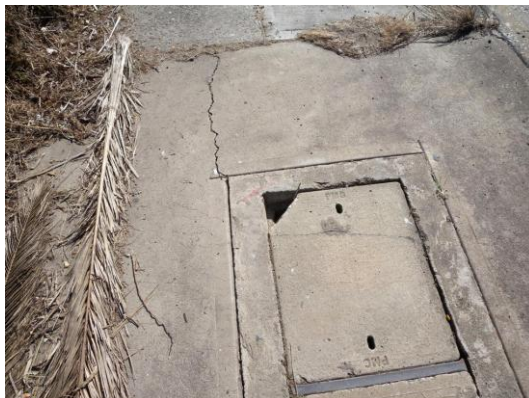
Figure 8.4: Damaged service pit in footpath
