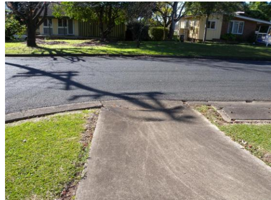
Figure 8.9: Unsatisfactory footpath repair with deterioration
