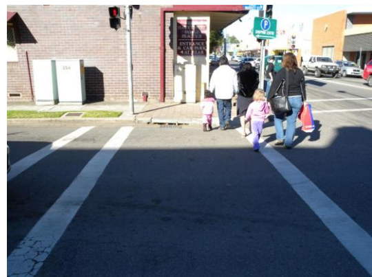
Figure 8.11: Narrow kerb ramps – pedestrians directed towards traffic
