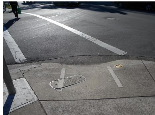
Figure 8.5: Kerb ramps at intersection – incorrect alignment
