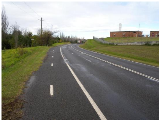
Figure 5.8: Unsatisfactory Intersection Linemarking
