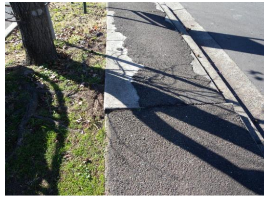
Figure 8.11: Narrow kerb ramps – pedestrians directed towards traffic
