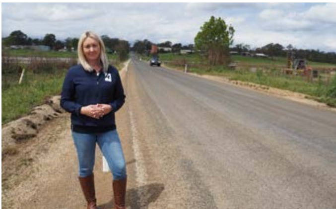
Road repairs at Wolseley Road, Oakville
