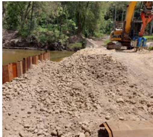
Upper Colo Bridge
