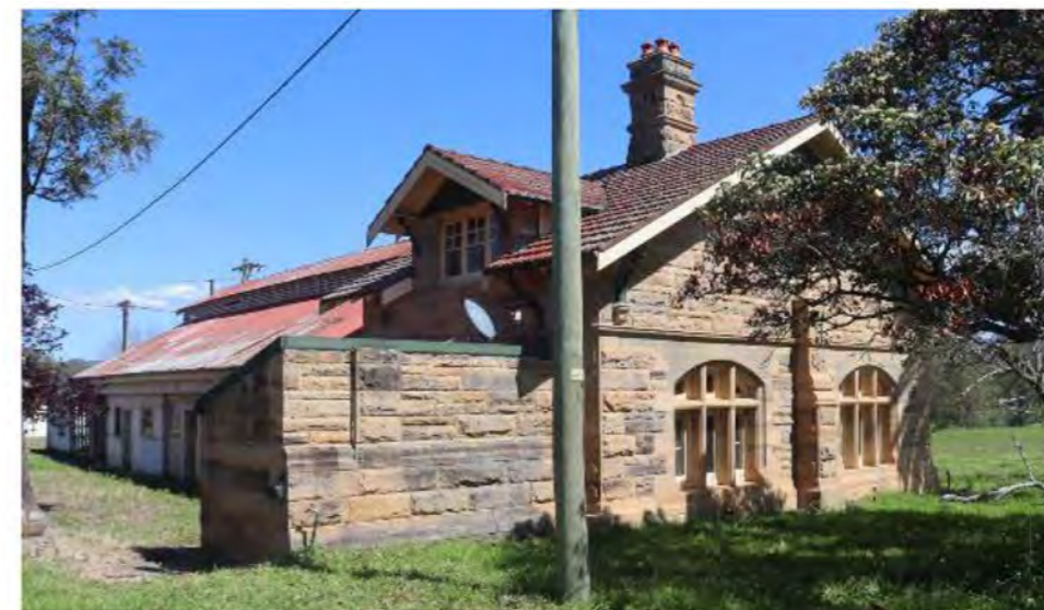
Plate 3-20: Building 2, looking south (AECOM, 2022)
