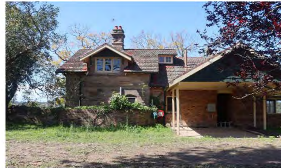
Plate 3-7: North western elevation of Building 1. This elevation faces building 2 (AECOM, 2022)
