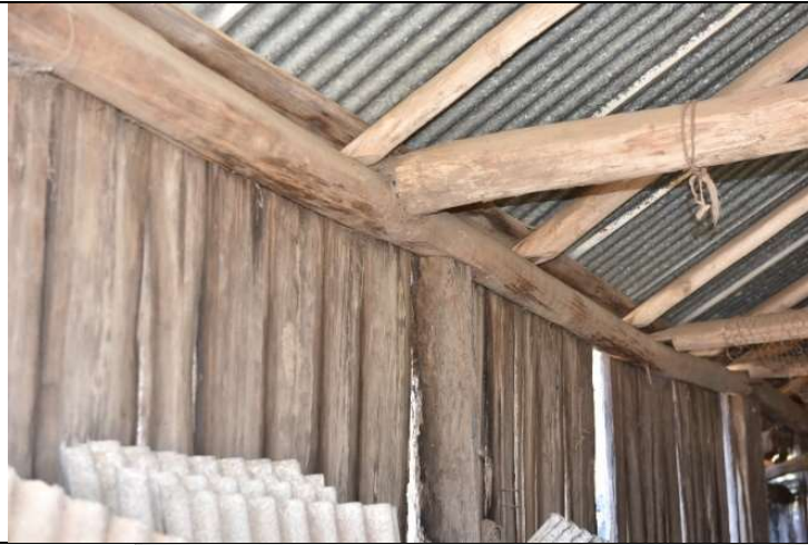
Caption: Detail of post/beam junction in barn at 1764 Upper Macdonald Road, Higher Macdonald Photographer: S. Johnson Copyright Owner: Lucas Stapleton Johnson & Partners Pty Ltd Date: June 2023
