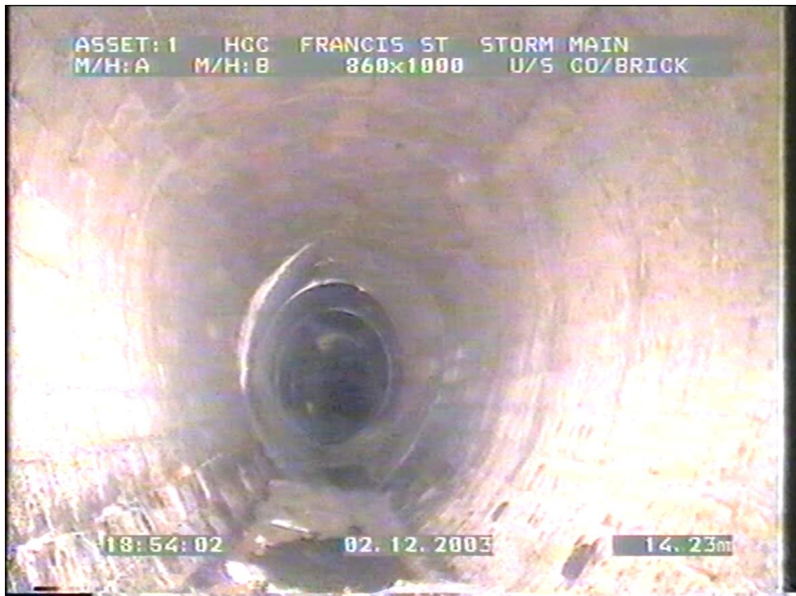
Photo 18 Interior of the brick barrel drain (Source: Hawkesbury City Council)
