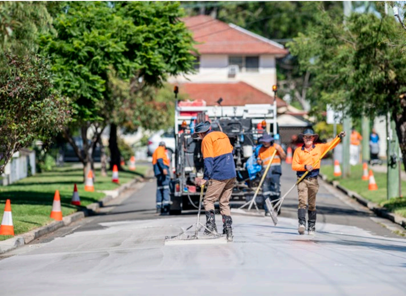
City of Parramatta installing heat-reflective coating as part of their Cool Roads Trial
