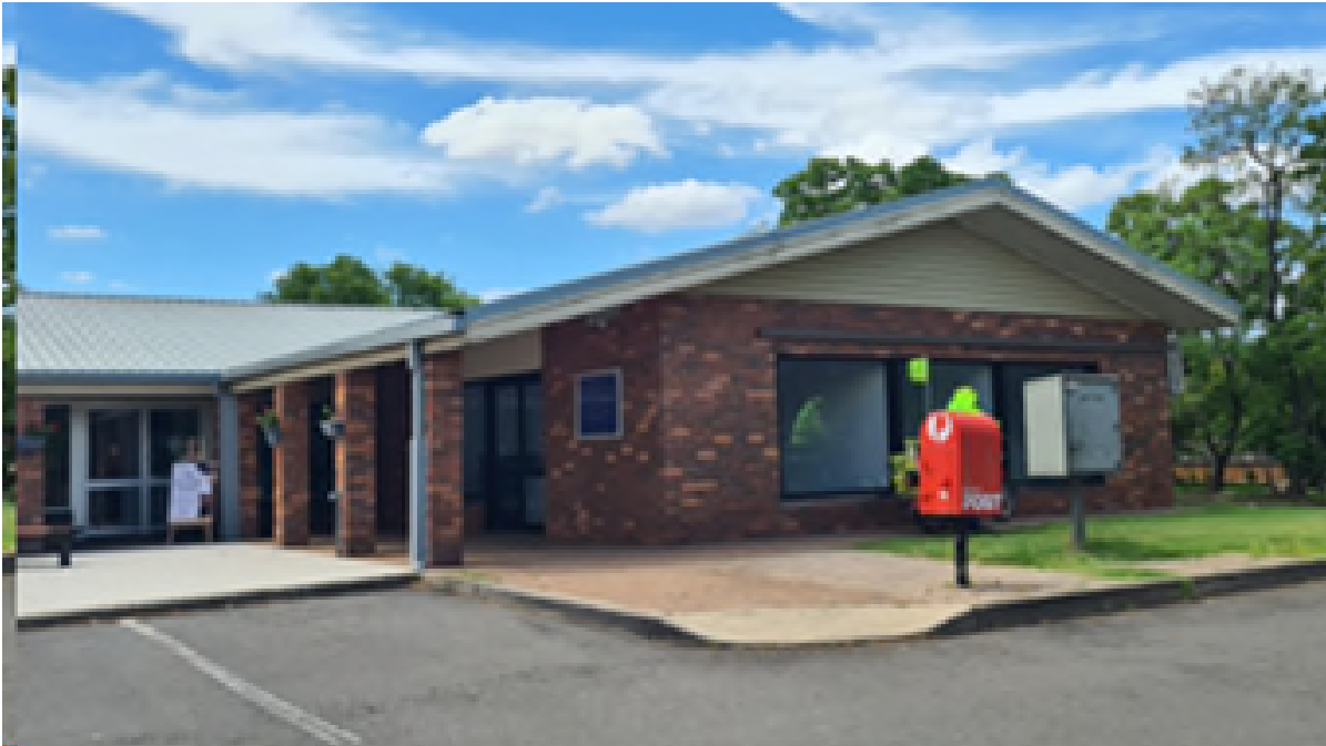
Figure 1 – Site photograph of the existing car park and shop frontage.
