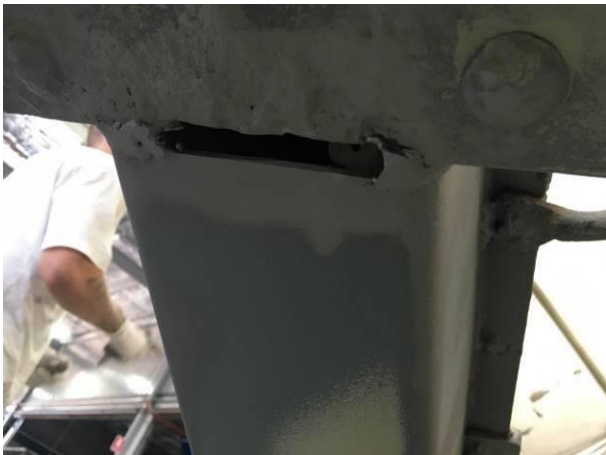
Figure 7 Creation of weep hole in trail
