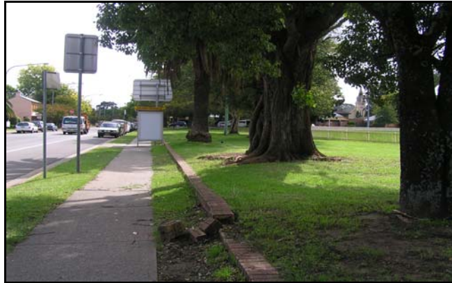
PHOTO 3: Richmond Park – view looking west along March Street frontage showing damaged brick edging (06/04/2009).
