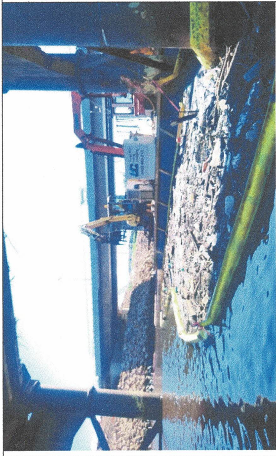
Fig. 5 – Removal of Accumulated Debris : Sothern Abutment
