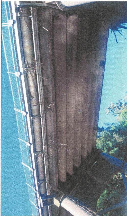
Fig.2 - Fourth Span from Southern Abutment: Entangled Debris
