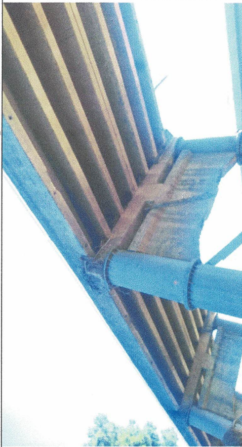
Fig.2 - Fourth Span from Southern Abutment: Entangled Debris
