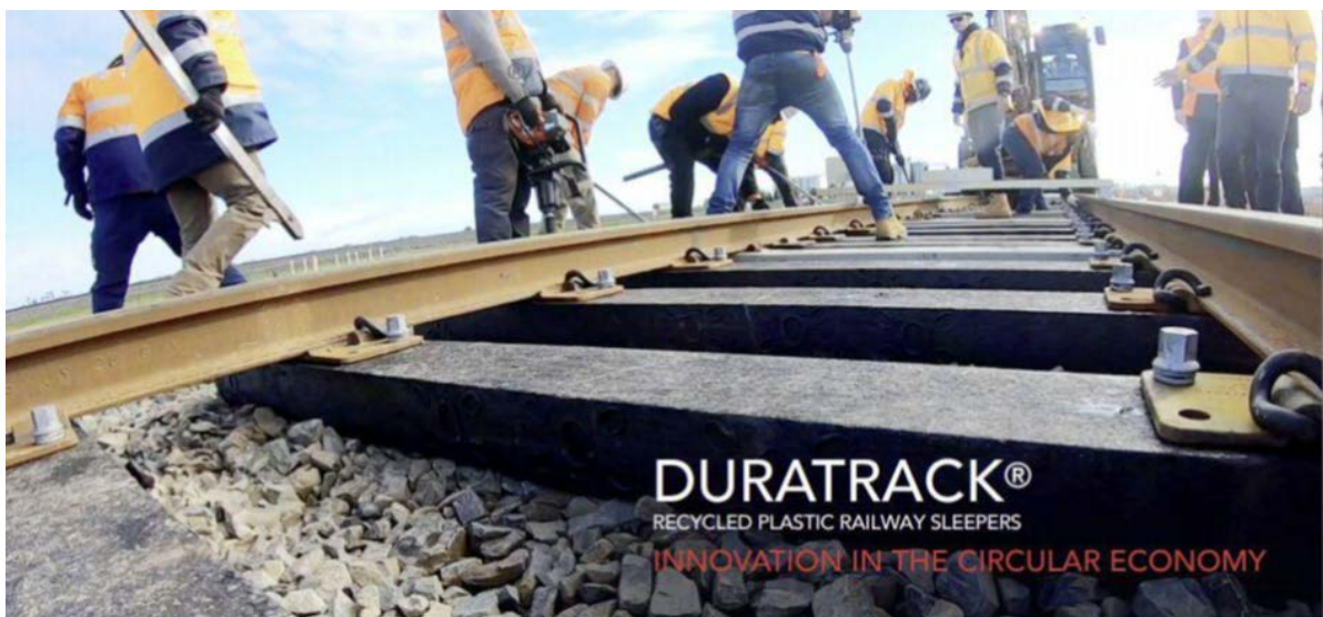
Image 1: Duratrack: Australia user of recycled densified EPS
