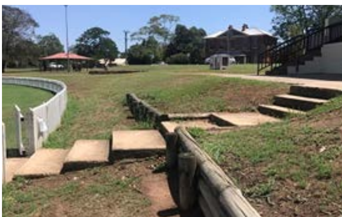
Photo 12: Slope between grandstand and oval showing erosion and poor seating options – refer to proposed works (3/02/2020).
