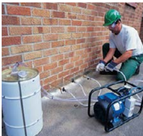
Figure 14: Chemical DPC impregnation in progress
