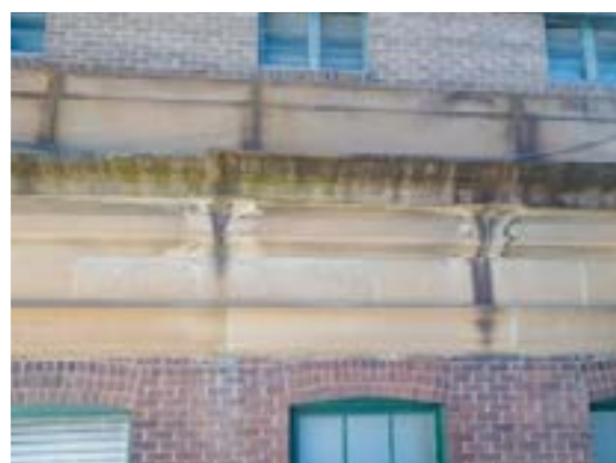
Figure 8: Open joints in cornice stones has allowed water with salts to discolour and damage stonework below
