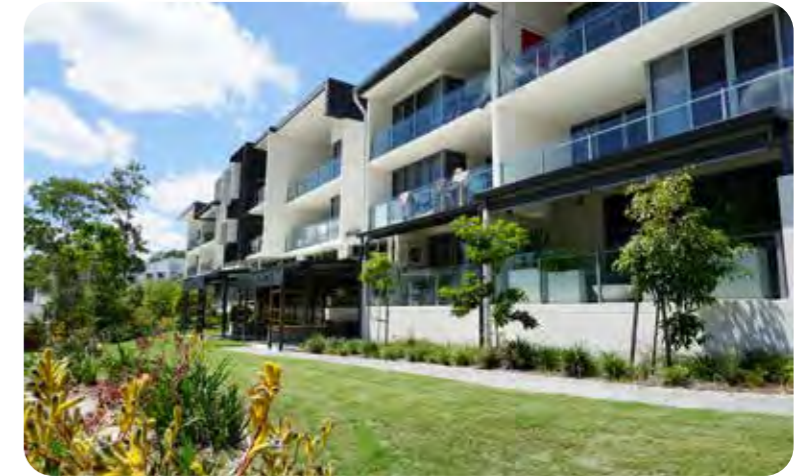
Apartments at Canopy, Bardon. Source: Tract
