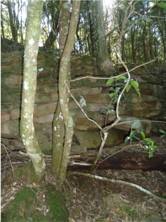
Plate 4: Trees growing within the mill race wall structure
