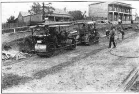
Fig. 1. Connecting road Windsor. Tractor towing roller.
