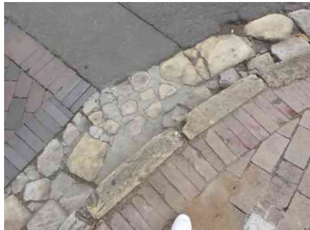
Figure 3. 114: Detail of sandstone kerb and edging with brick footpath paving at the junction of George Street and Thompson Square.
