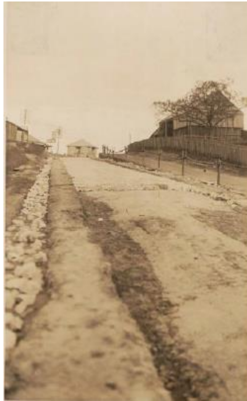
Photo 39 1924 photograph of reconstruction of the main road in Windsor (Source: (State Library of NSW, image no. 2024-a038-001671, cited in AAJV 2017)
