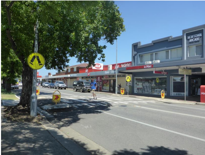
Photo 13 Example of paved footpaths, signage, traffic management infrastructure, concrete kerbs and gutters and sealed roads
