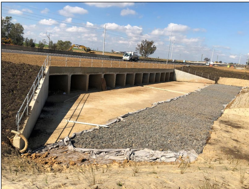
Figure 30 Multi-cell box culvert under construction
