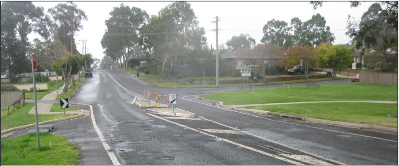
Figure 16 Pedestrian refuge, Wollondilly Shire
