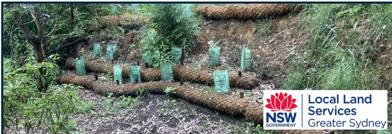
Erosion control and bank stabilisation using coir logs
