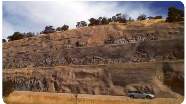
Shotcrete applications extend neatly to the edge of a change in the rock surface and coloured to match existing rock can look quite unobtrusive and visually acceptable. (Southern Freeway M1.)
