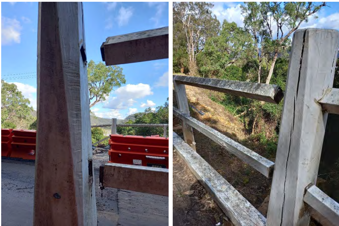
Figure 3-21: Views of damaged timber elements of the bridge. (Source: OCP Architects, August 2022.)
