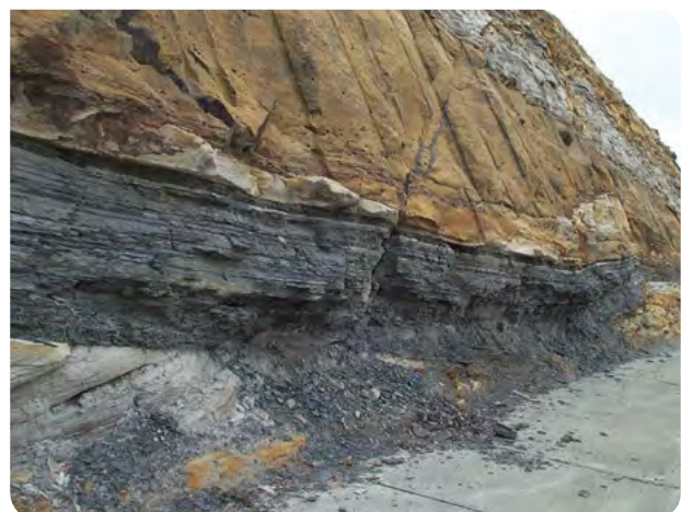
A crumbly shale band, which if higher up the cutting would need to be stabilised.
