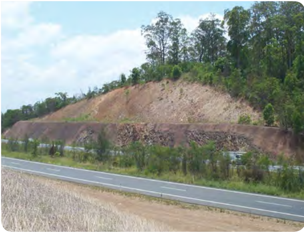
A dark earthy red/grey/brown colour helps recede the shotcrete into the rock of the lower half of the cutting on the Pacific Highway near Taree.
