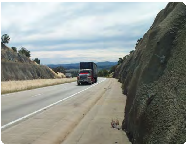
Two cuttings on Hume Highway, one with a setback and limited shotcrete (left), the other adjacent to the road requiring significant shotcrete coverage.
