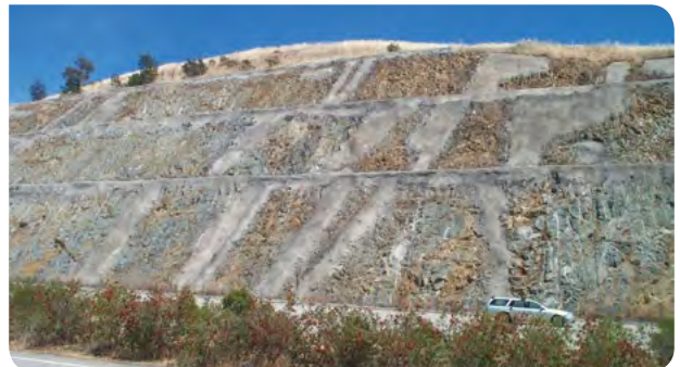
Two cuttings with similar stability problems. Precision design and progressive stabilisation can minimise the extent of shotcrete (Hume Highway).
