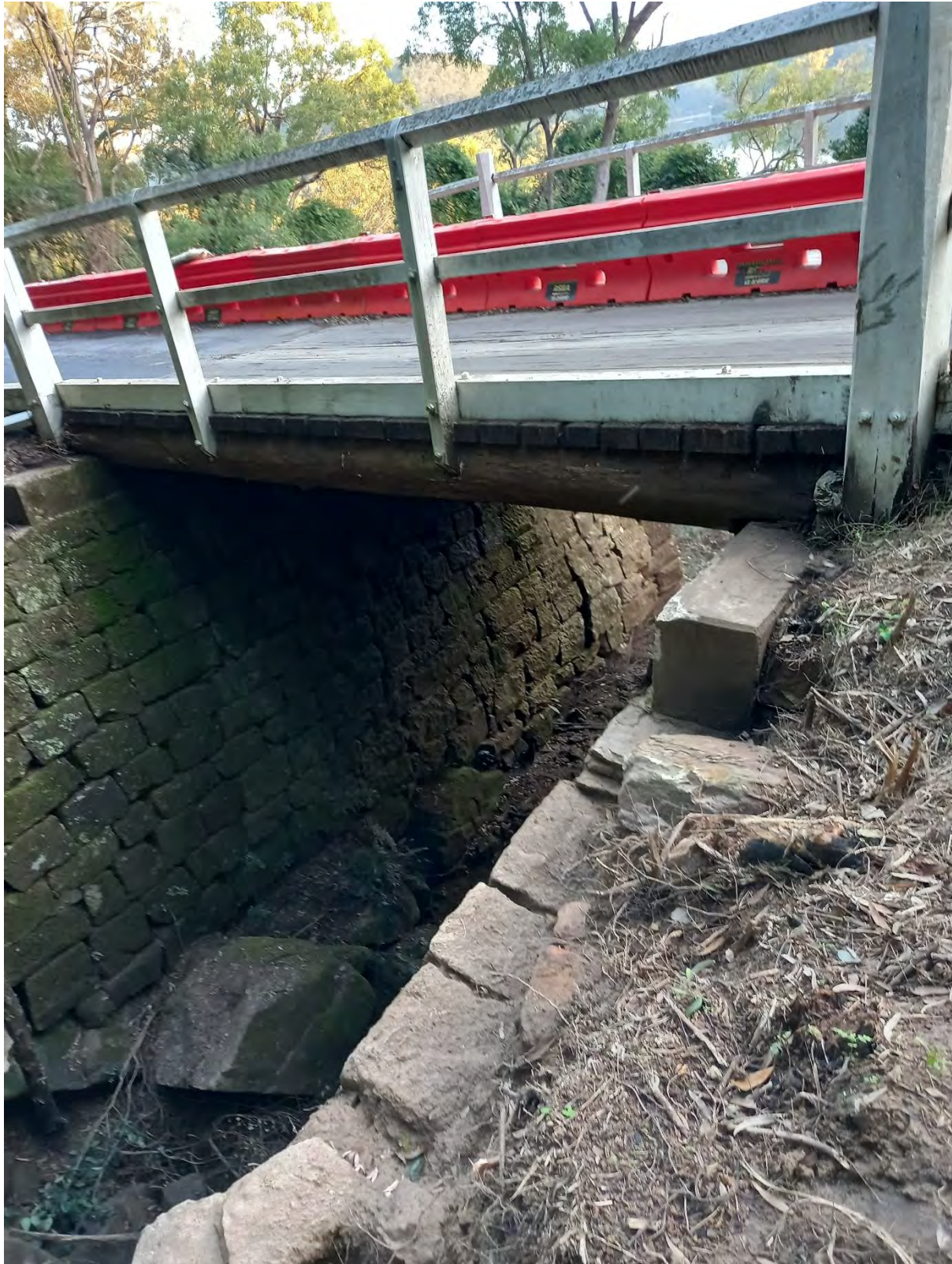
Figure 3-15: View of the bridge and the stone-lined channel underneath. (Source: OCP Architects, 2022.)
