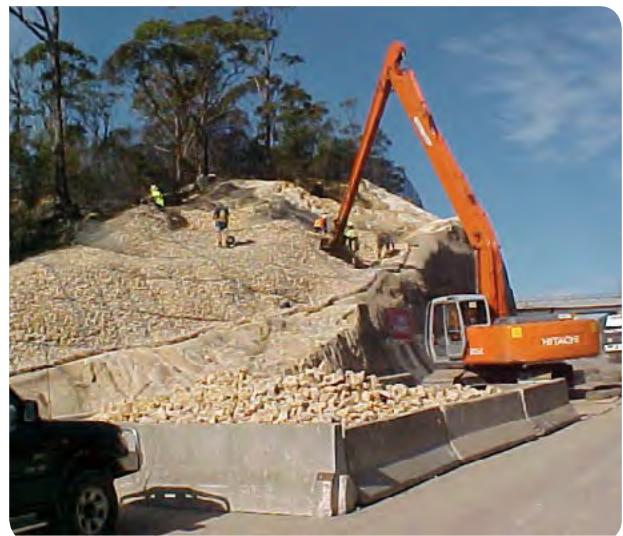
Rock filled mattresses placed over shotcrete application, Great Western Highway at Linden.
