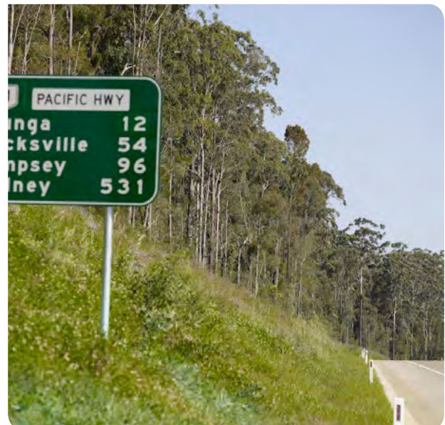
A vegetated 2(H):1(V) cutting on the Pacific Highway at Bonville providing a long term outcome.
