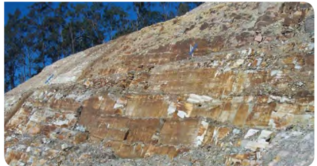
The natural jointing of rock often creates a texture which is angular and planar rather than amorphous, so unformed shotcrete does not complement this well and has a poor appearance (picture above).
