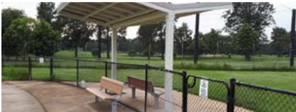
New shelter for Pound Paddock off-leash area at Richmond.
