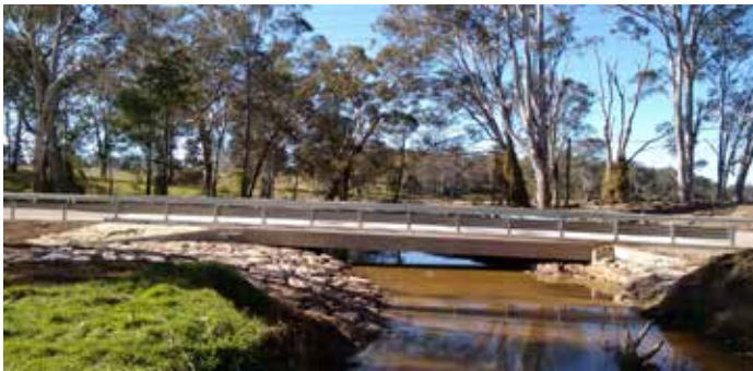
West Portland Road Bridge, Lower Portland
