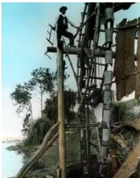
Water pump on the river near North Richmond Bridge, date unknown. Hawkesbury Library Service.
