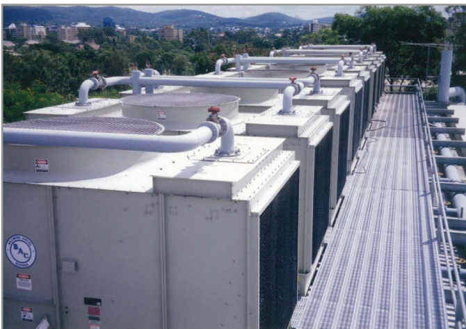
Figure 5.2-2: Cross-flow cooling towers with rectangular covers at the top of the towers (preventing entry of sunlight) and a walkway for safe and easy access
