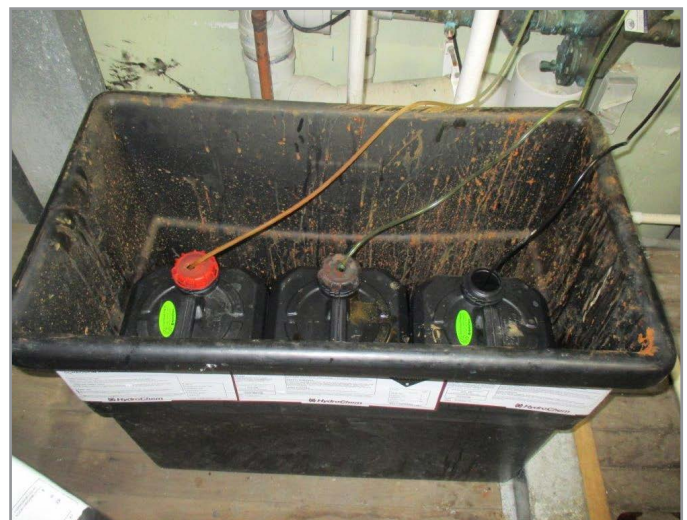
Figure 5.3-5: A bund container that may compress dosing tubes when the lid is replaced
