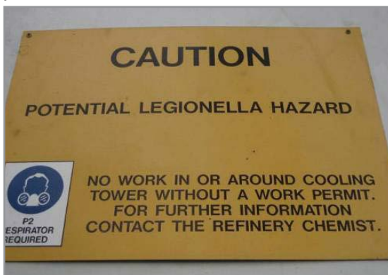
Figure 5.5-1: Signage provided at a cooling water system premises
