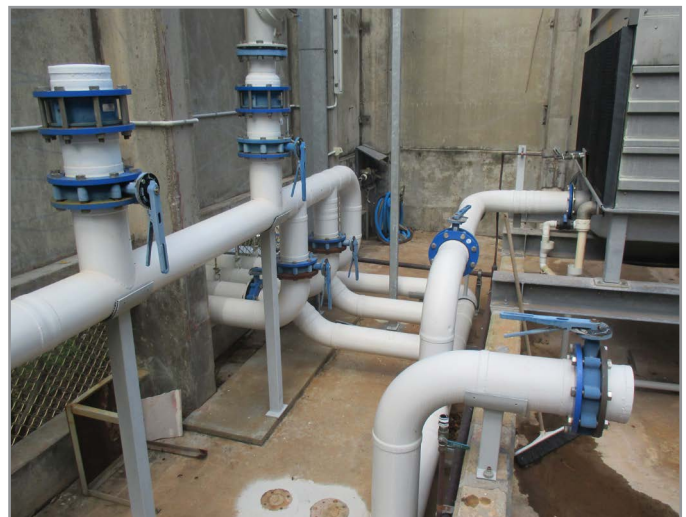
Figure 5.1-1: Two dead legs (top left and bottom right)
