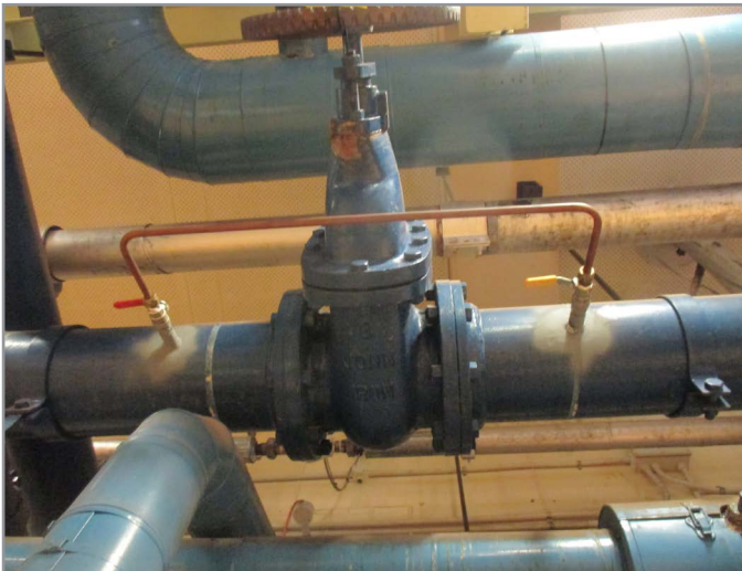
Figure 5.1-2: Solution for managing dead legs (small-bore bypass)
