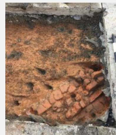
East-facing view of the sandstock brick box drain Test Pit SA26 (AAJV
