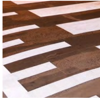
Windsor Street upgraded pedestrian crossing
