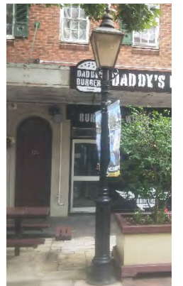
George Street Pedestrian Mall existing gas lamp
