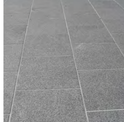
George Street paving - Dimensioned Paver (600 x 300mm)
