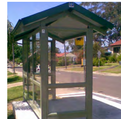
Bus stop upgrade along George Street
