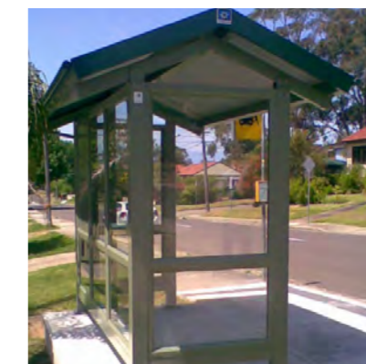
Bus stop upgrade along George Street
