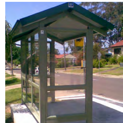
Bus stop upgrade along Windsor Street
