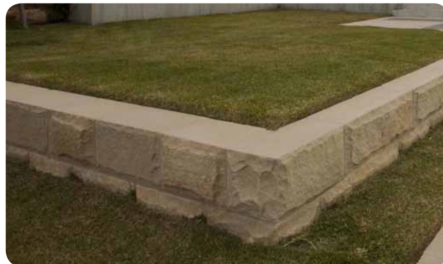
Sandstone retaining sitting wall to levelled stage area
