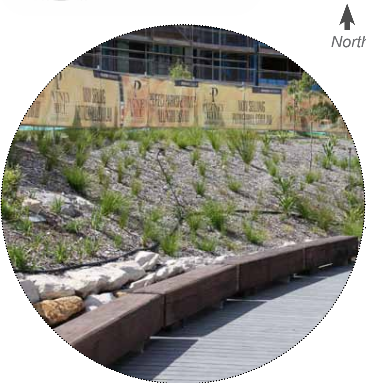
Recycled timber sleeper bench seat
