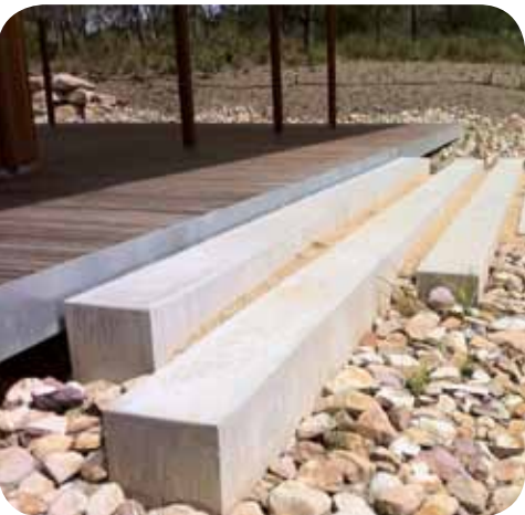
Concrete sleeper steps with gravel infill
