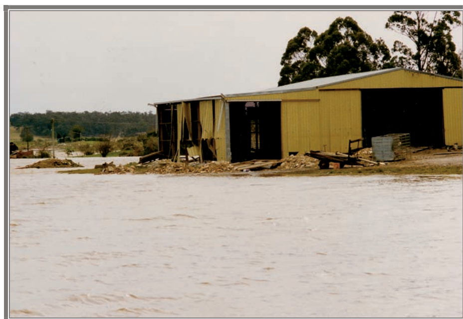
FIGURE 2.2 – Damage to Shed opposite Butterfly Farm, Wilberforce, August 1990 Flood, Attributed to Waves
