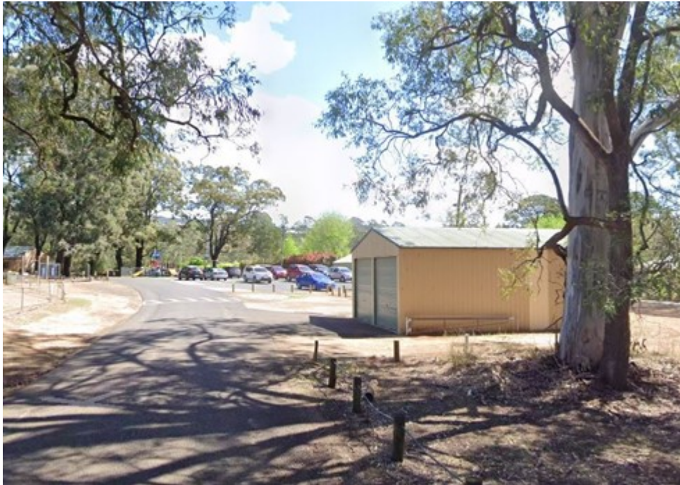
Figure 2 – Existing Bus Shed, McMahon Park, Kurrajong
