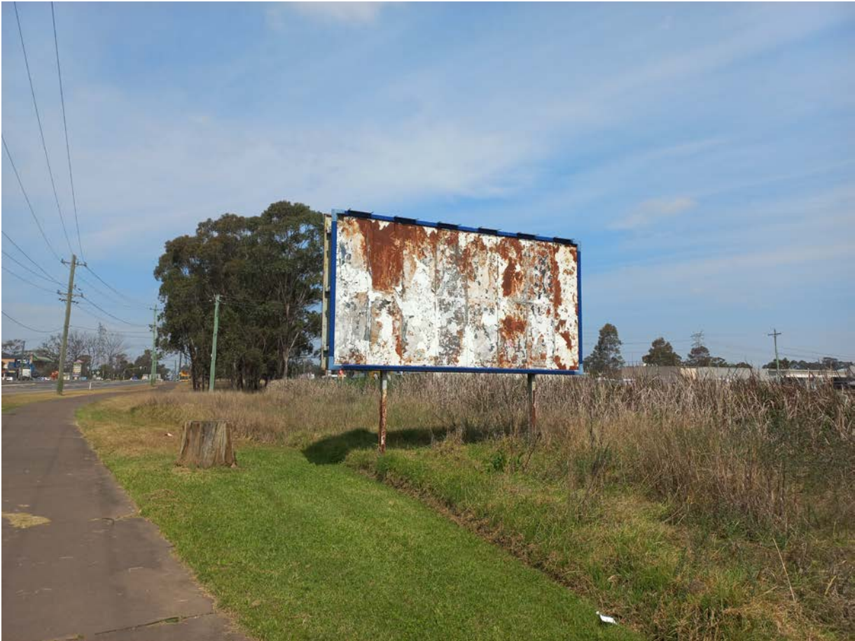
Figure 8. Rear of existing billboard sign.
