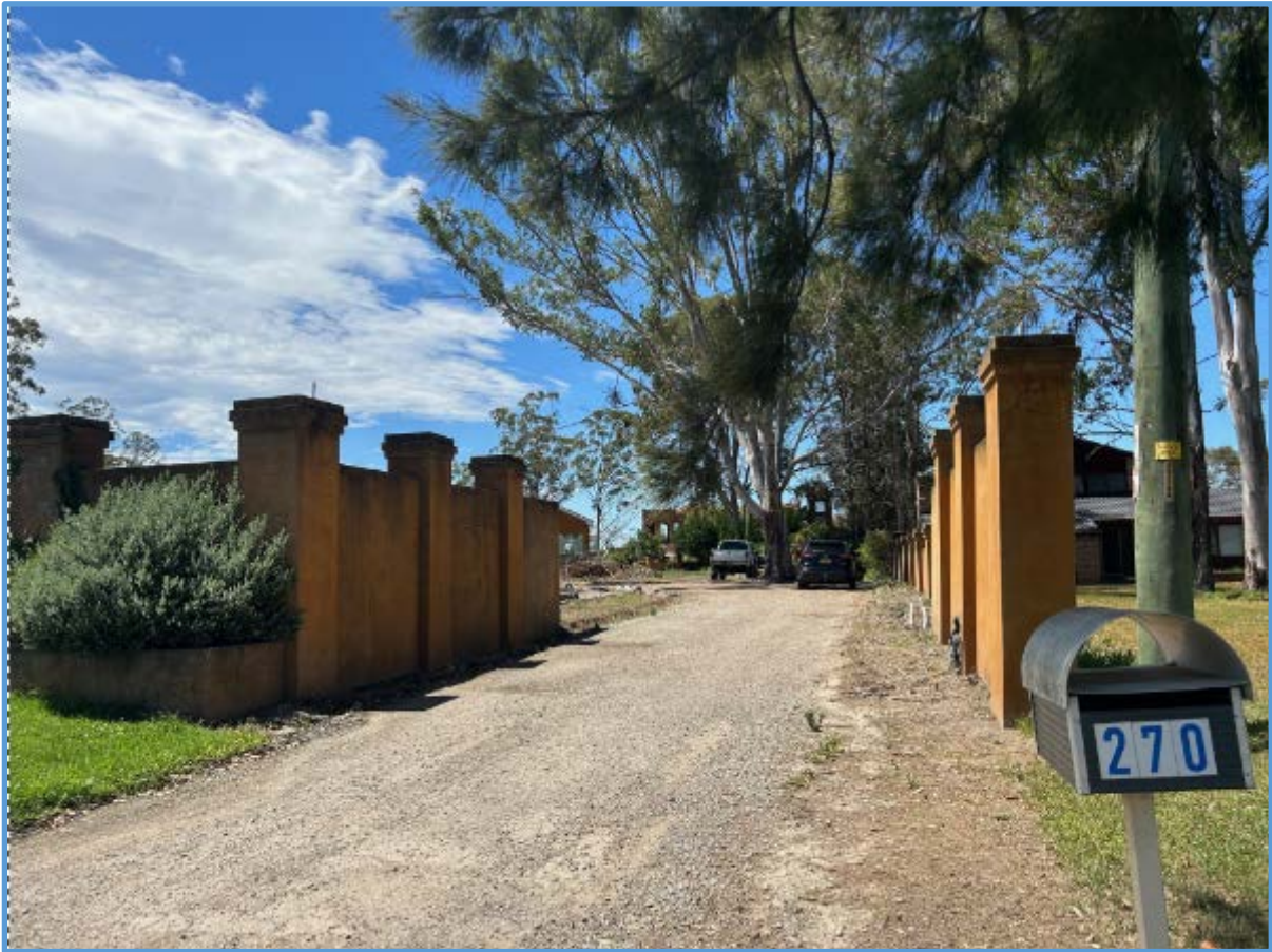
Figure 8: 270 Terrace Road, North Richmond looking south from Terrace Road.
