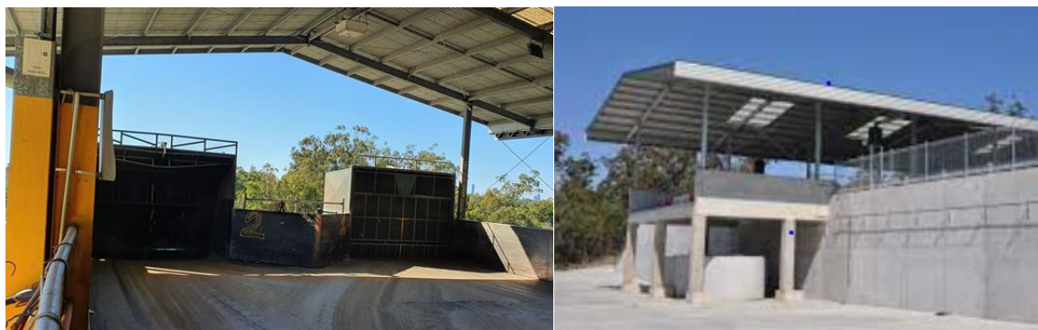
Figure 4: Shallow push pit floor to the left and backdrop into the compactors to the right at Molendinar (City of Gold Coast).
