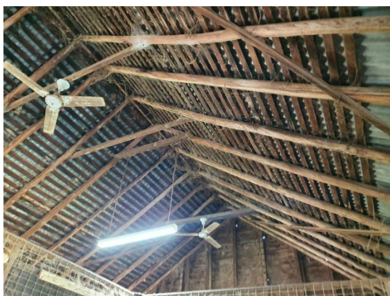
Figure 3. 26: Barn 2 'Bottom stables' at Hobartville, No.36-40 Inalls Lane, Richmond with pole rafters and shingle battens.
