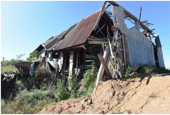
Figure 6. 3: Early 19 th century slab barn at No. 56 Freemans Reach Road, Freemans Reach showing the impacts of 2022 floods on the structure as a result of the washing away of river bank.
