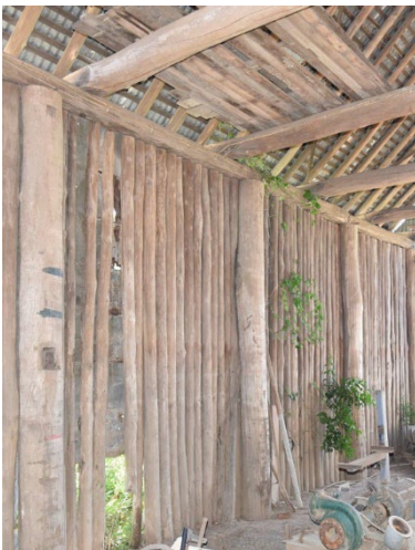
Figure 3. 28: Detail of palisade wall cladding and shingle battens to barn at No 56 Freemans Reach Road, Freemans Reach.
