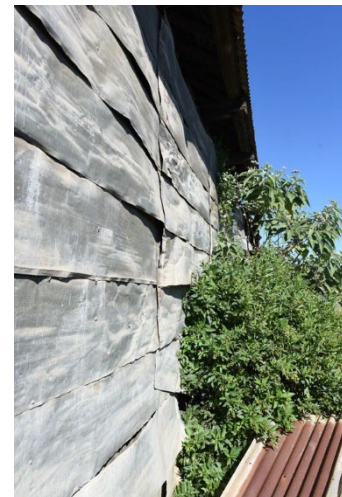
Figure 3. 30: Flat iron plates covering over original wall cladding to barn at No. 56 Freemans Reach Road, Freemans Reach.
