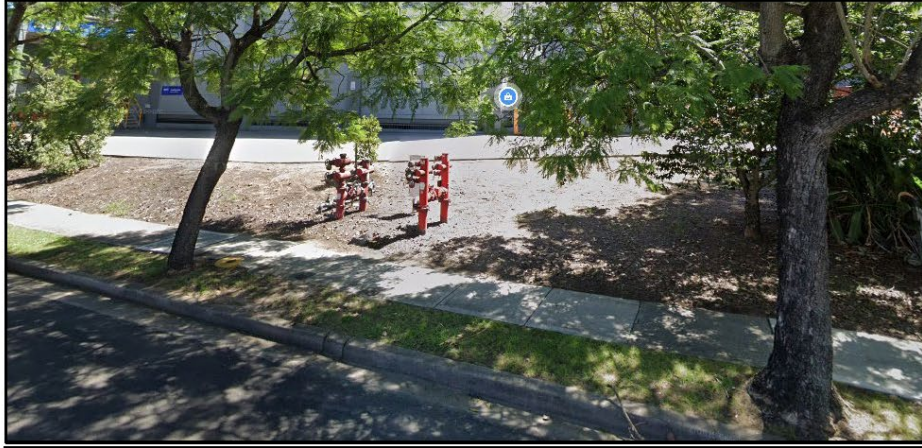
Street view image of the hydrant booster assembly at the Lennox Street entrance to the property Source: Google Maps – Feb 2025
