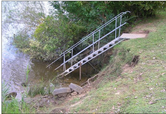
PHOTO 11: Privately constructed metal steps/ handrails on eroded riverbank. Concrete rubble and tyres along water's edge (5/04/2012).
