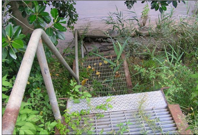
PHOTO 10: Damaged private metal-grille steps/ handrail on eroded riverbank. Broken concrete rubble platform and tyre wall (22/03/2013).
