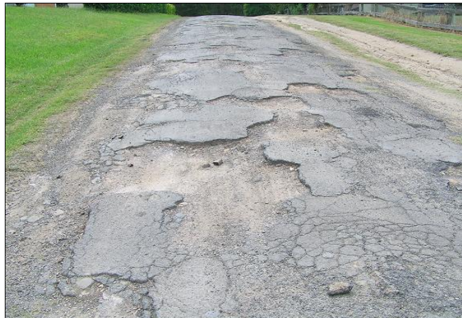
PHOTO 6: Bitumen road surface (public access road into reserve) is in need of urgent repair (LandArc image 22/03/2013).
