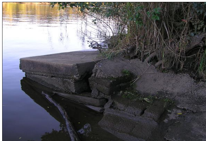
PHOTO 26: Boat launching ramp – ad hoc armoring to adjacent walls. Ramp conditions pose public safety risks, particularly at high tides/ fast river flows (LandArc image 27/05/2012).
